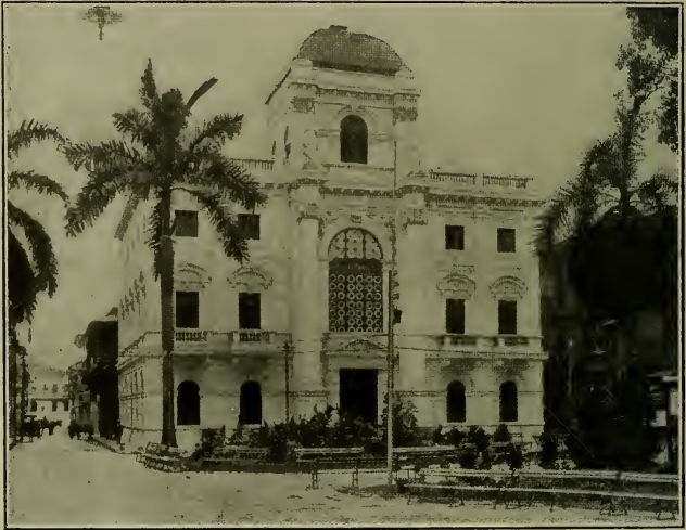
NEW PANAMA CITY MUNICIPAL BUILDING, PLAZA INDEPENDENCIA.
