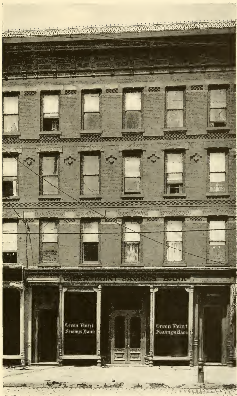
TEMPORARY QUARTERS AT 127 GREEN POINT AVENUE
