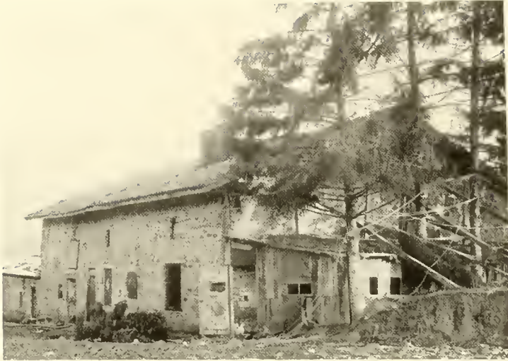
On the edge of the Argonne Forest—building at LA BESOGNE used as a Command Post.
