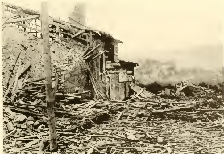
Dwellings on the outskirts of GRAND PRÉ suffered same as those in the town proper
