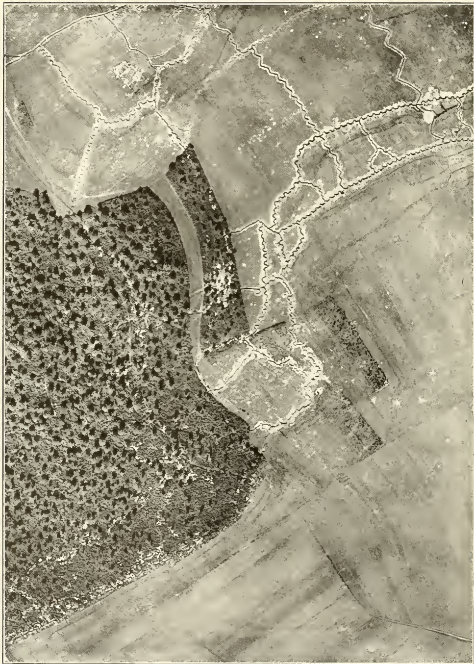
German--built trenches in the woods and in the open, part of Hindenburg Line N. W. of LIMEY, France--note the numerous shell holes. Air photo, taken August 25, 1918, noon, at height of 3,000 meters
