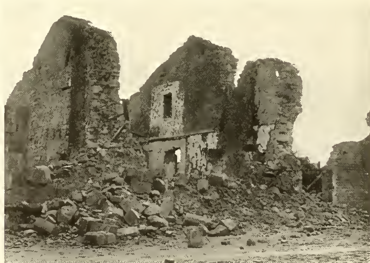
These massive thick walls at CHEVIERES crumpled under the heavy artillery pounding
