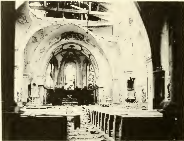
Interior of THAUCOURT Church
