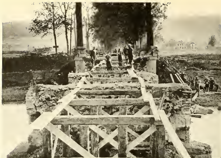
Under almost constant enemy fire, our 303rd Engineers repaired necessary bridges over the Aire River.
