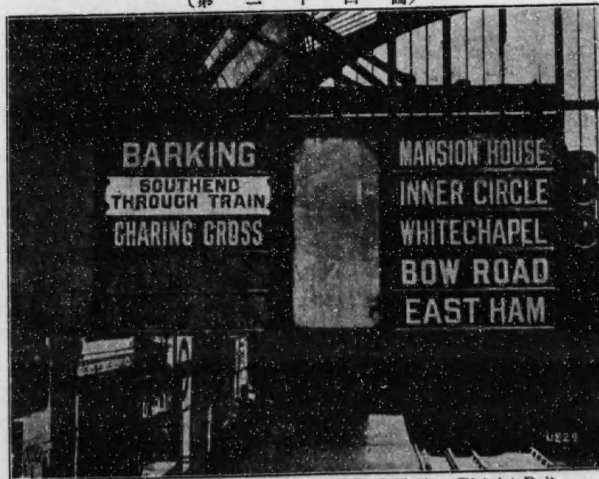
Fig. 24. — Destination indicator, St. James' Park Station, District Railway.
