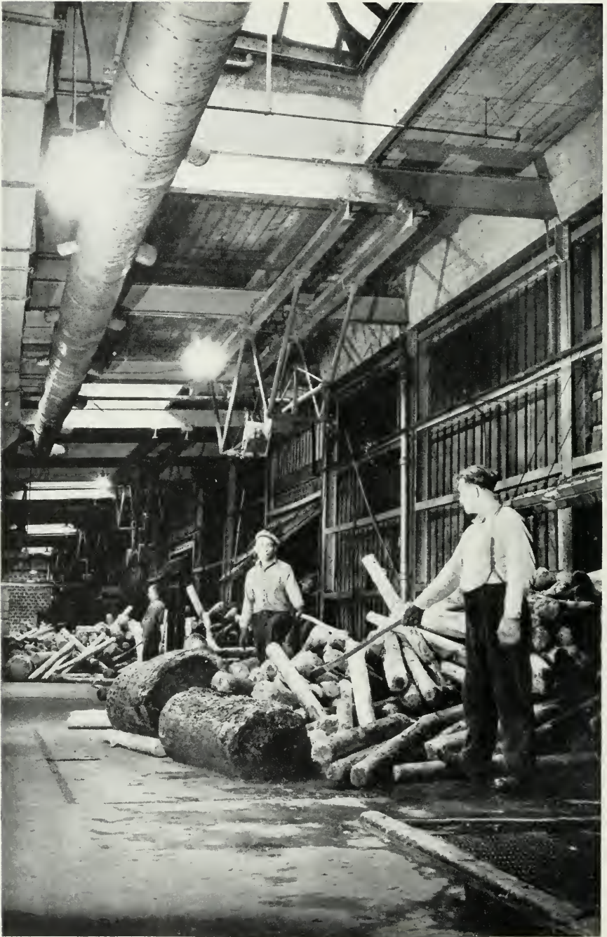
CHARGING FLOOR AT GROUND WOOD MILL
