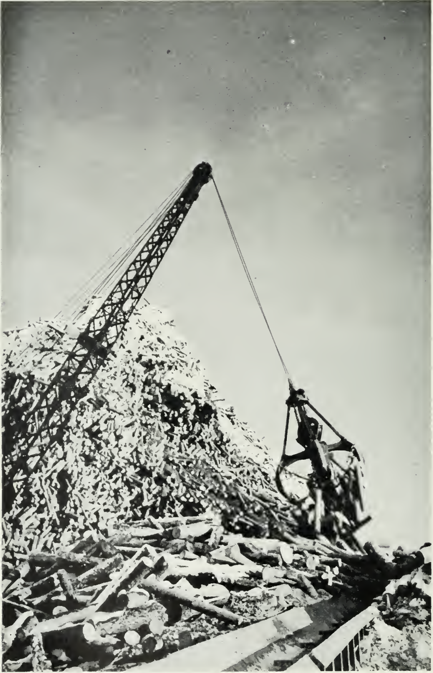
A DIESEL GRAB DROPPING PULP ONTO BELT
