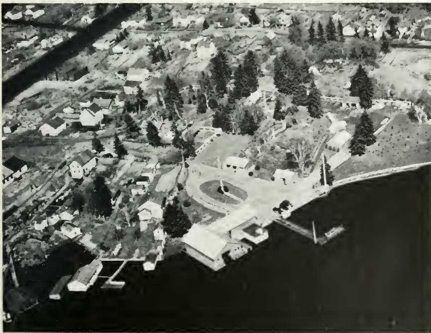
AERIAL VIEW OF CHIEF RANGER'S HEADQUARTERS, KENORA
