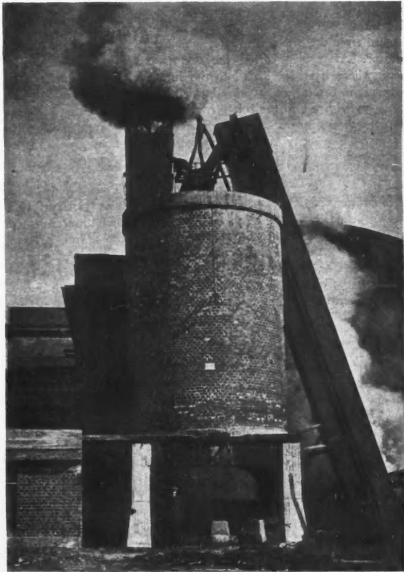
DRYING PLANT AT J. W. ENQUIST, AB., TAMMERFORS, CAPACITY 10,000 CUBIC FEET PER 24 HOURS
