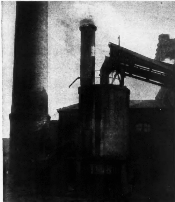
DRYING TOWER AT VÄSFERVIK, CAPACITY 5,000 CUBIC FEET PER 24 HOURS
