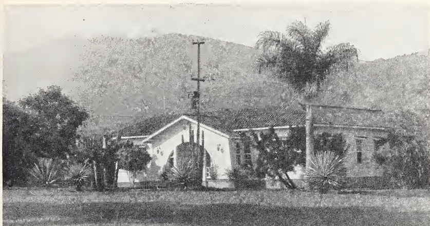
FIGURE 2.—Office and laboratory of the United States Department of Agriculture at the cooperative rubber plant field station near Turrialba, Costa Rica.
