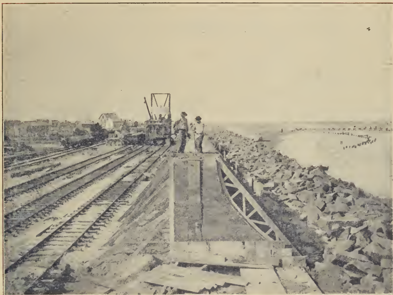
View Looking East Showing Seawall, Riprap and the Gulf.
