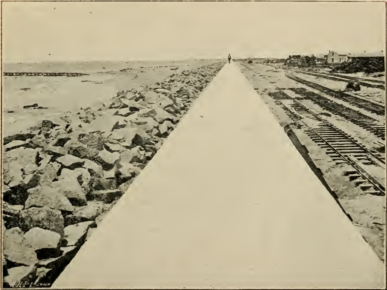
View from Top of Seawall, Looking South, Showing Bend in Seawall.
