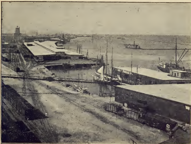
Wharf Scene, Looking West.
