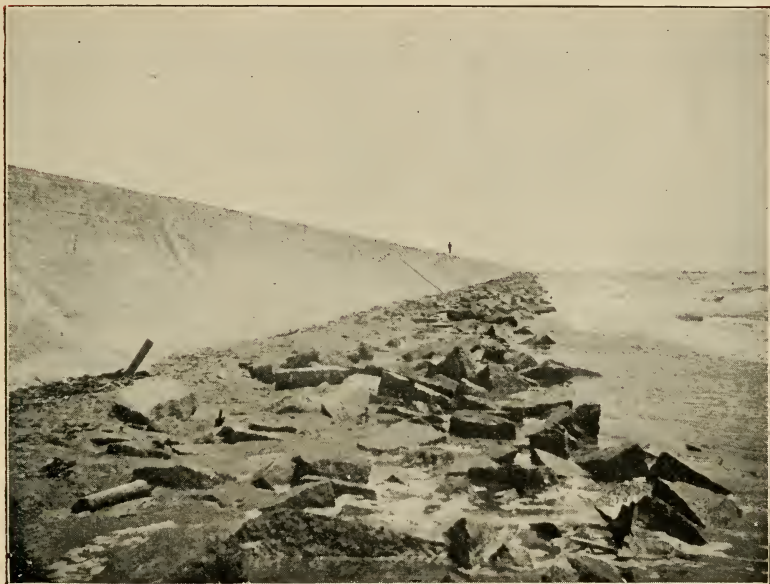
View of Seawall, Looking East.
