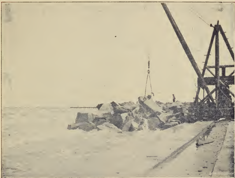
Foundation of Seawall and Placing the Riprap.
