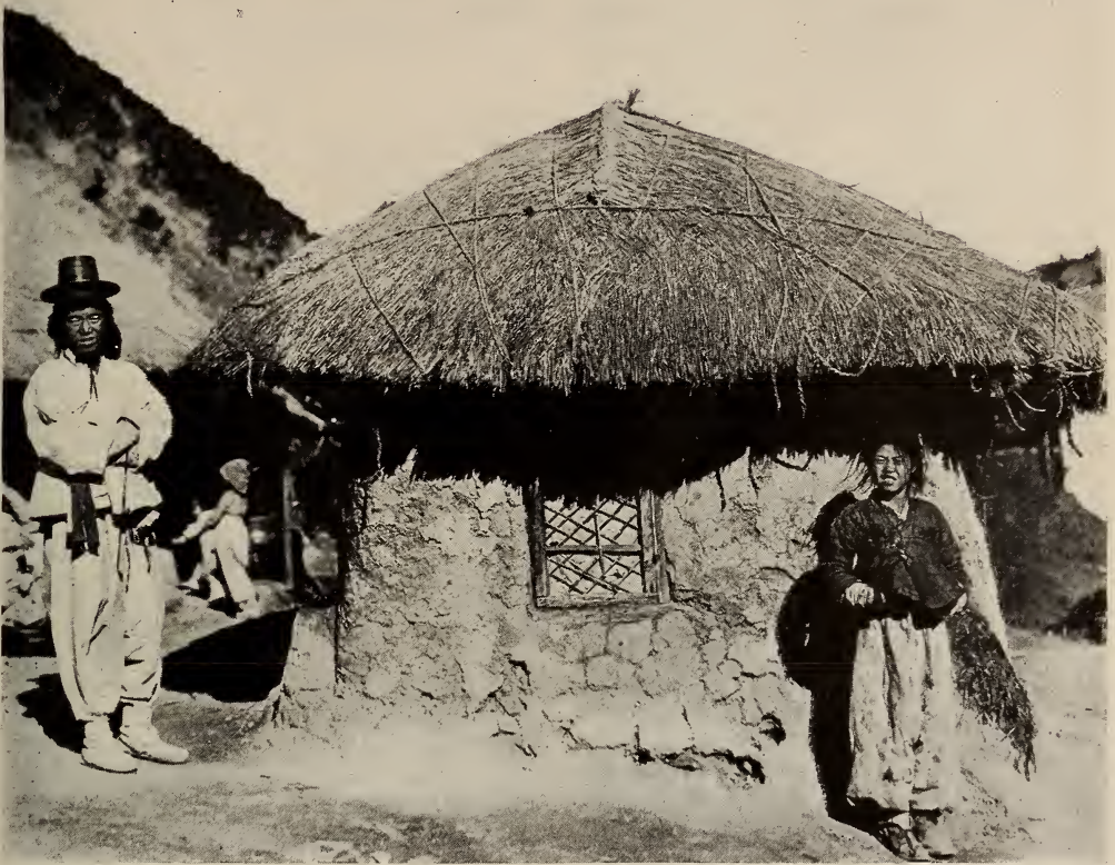
THE WALLS AND FLOOR OF THIS TYPICAL NORTHERN KOREA HOUSE ARE MADE OF CLAY; THE THATCH IS OF RICE STRAW
