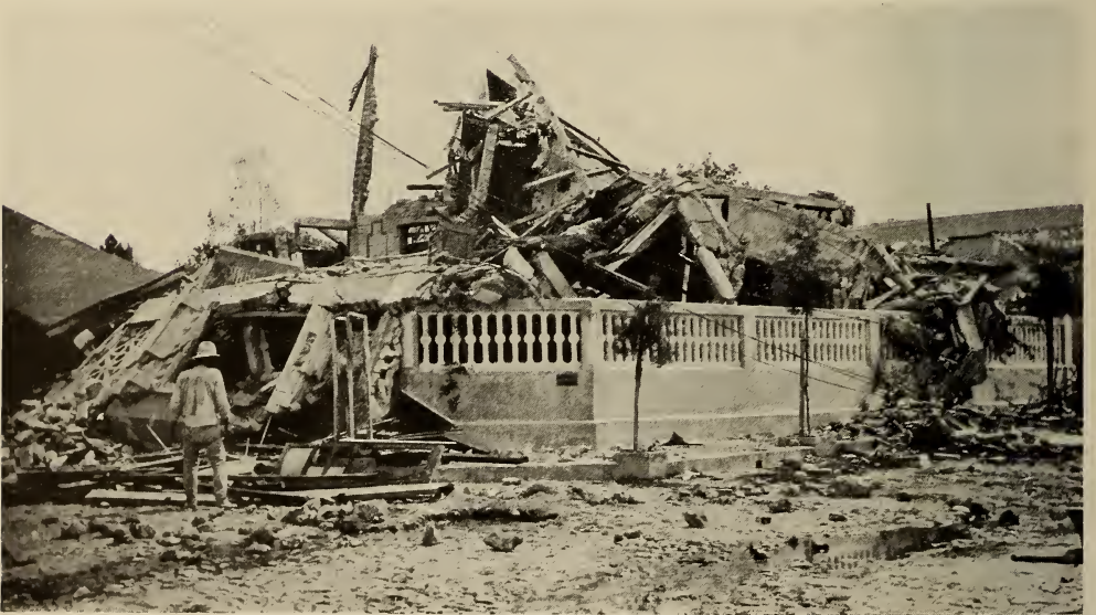
A HOUSE OF LIGHT CONCRETE CONSTRUCTION REDUCED TO A PILE OF DEBRIS BY THE EARTHQUAKE: SAN SALVADOR
