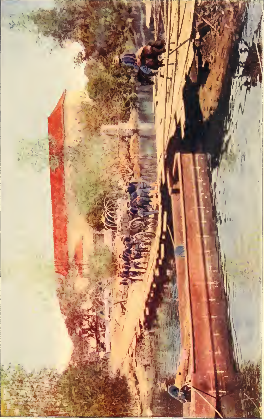
The engineers were adept at making pontoon bridges over which the heaviest artillery and ammunition wagons could be taken with safety. This bridge is across the Bigaa river and the wagons are being hauled by men from lack of draft animals
