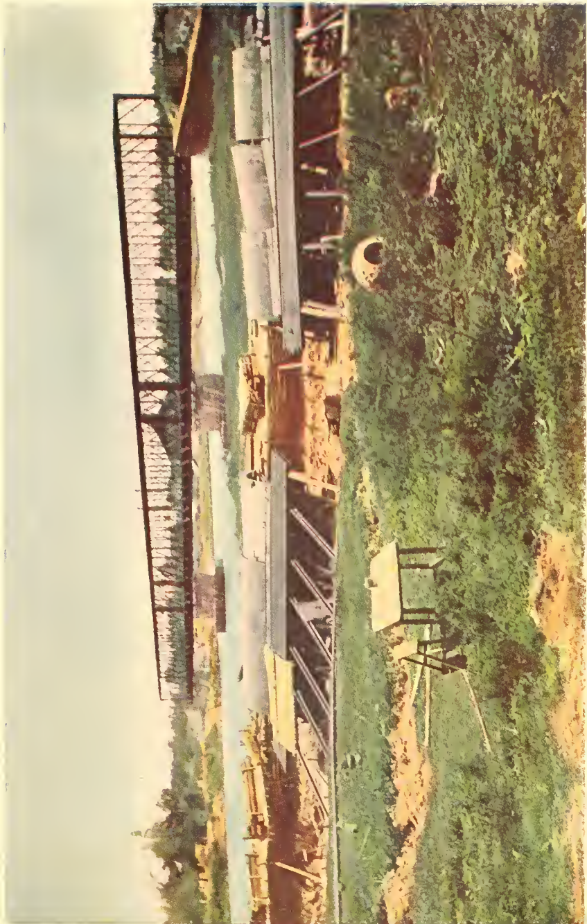
CALUMPIT.—The steel railroad bridge seen here, with its barricaded entrance, was fortified by the insurgents to prevent the crossing of the American troops during advance on Malolos. It was captured by Funston, who crossed the river with sixteen men and routed the insurgents, with great loss to them.
