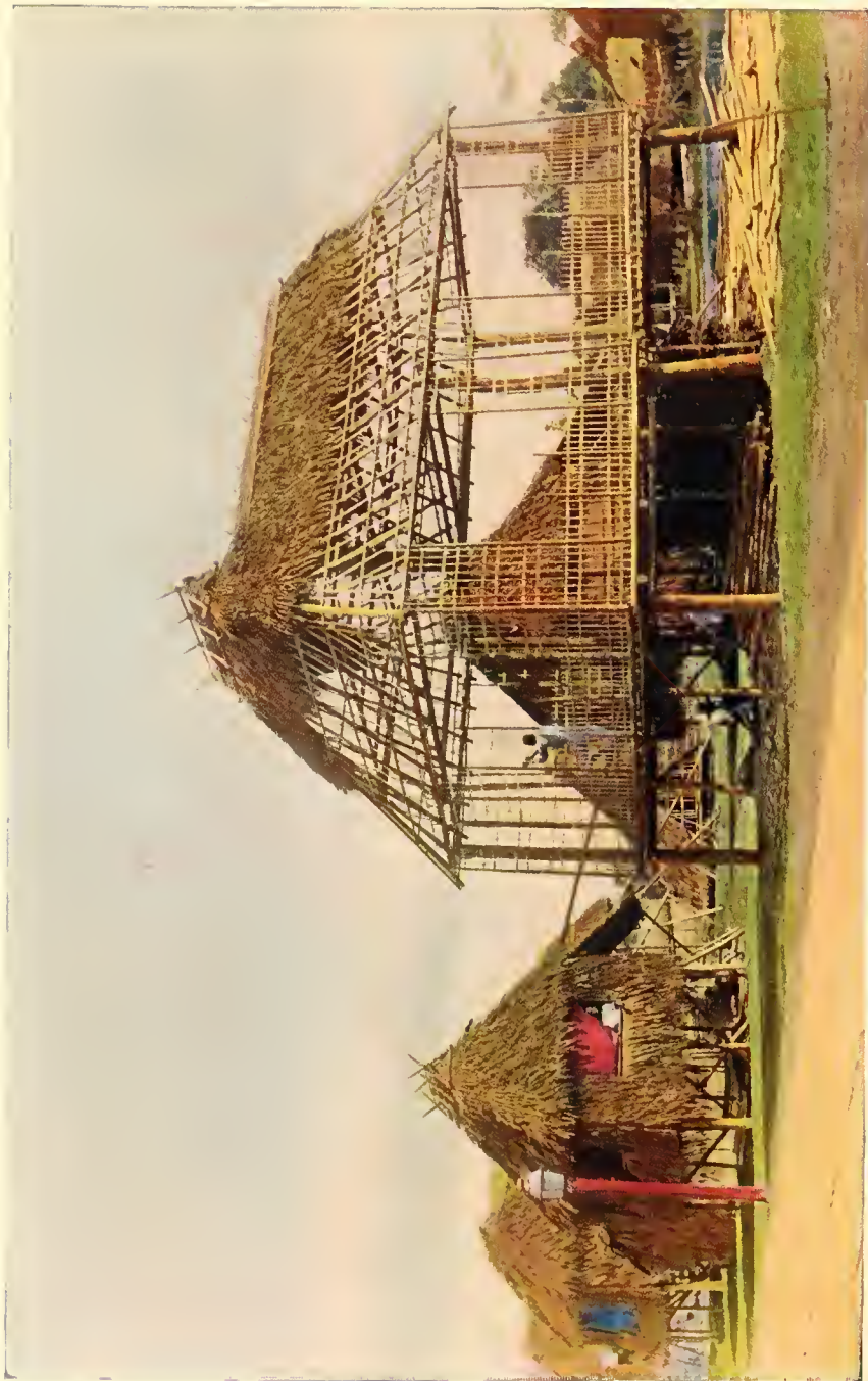
The houses of the natives in the interior are built as seen here to provide against both flood and earthquake. In this view the mode of construction may be seen. The roof is the first part to be woven in after the frame is made.
