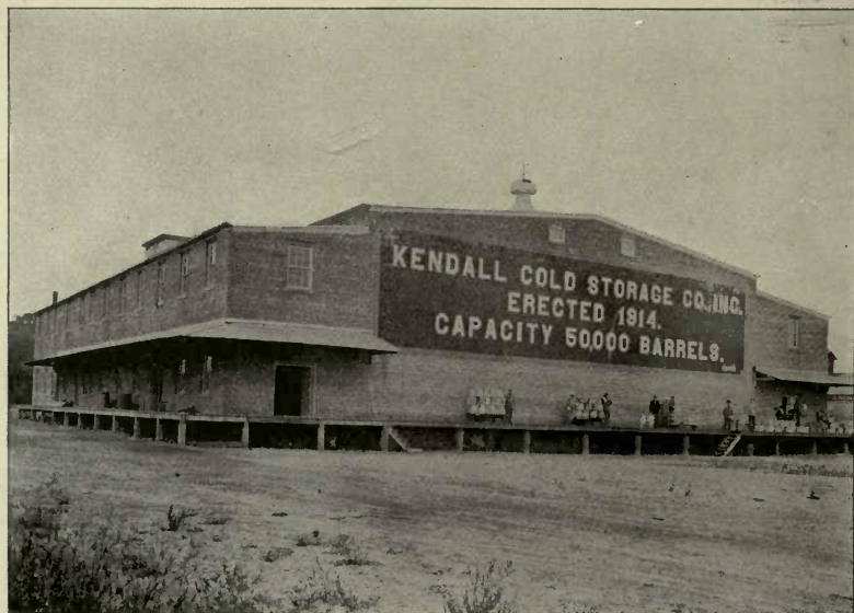
FIG. 170.— COLD STORAGE HOUSE AT KENDALL, ORLEANS COUNTY (Courtesy of Kendall Cold Storage Co., Kendall, N. Y.)
