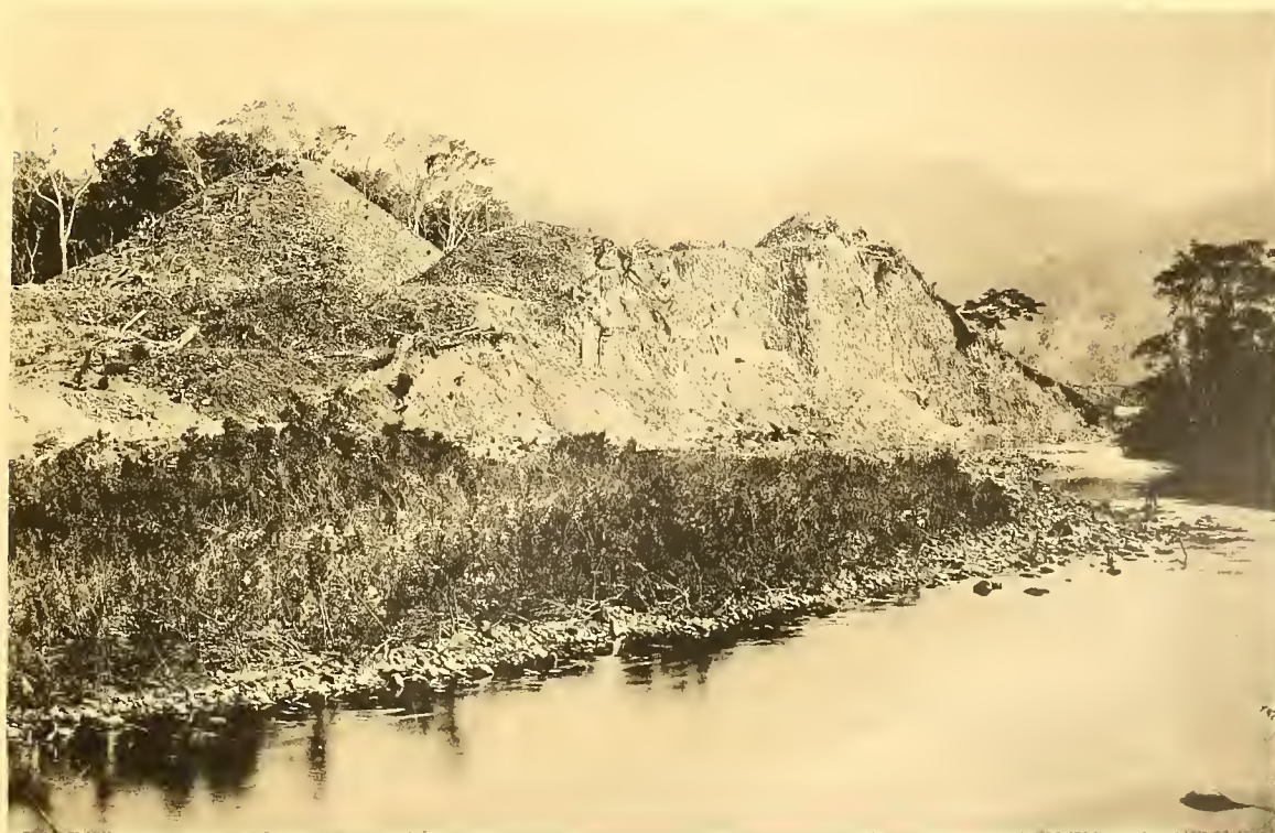
b. The main structure looking northwest.
