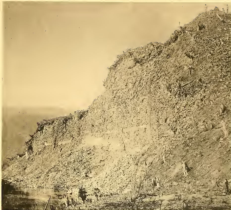
a. The main structure looking southwest, showing the great cross-section exposed by the river.
