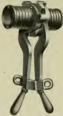
THE CURTIS AUTOMATIC PIPE COUPLING.
