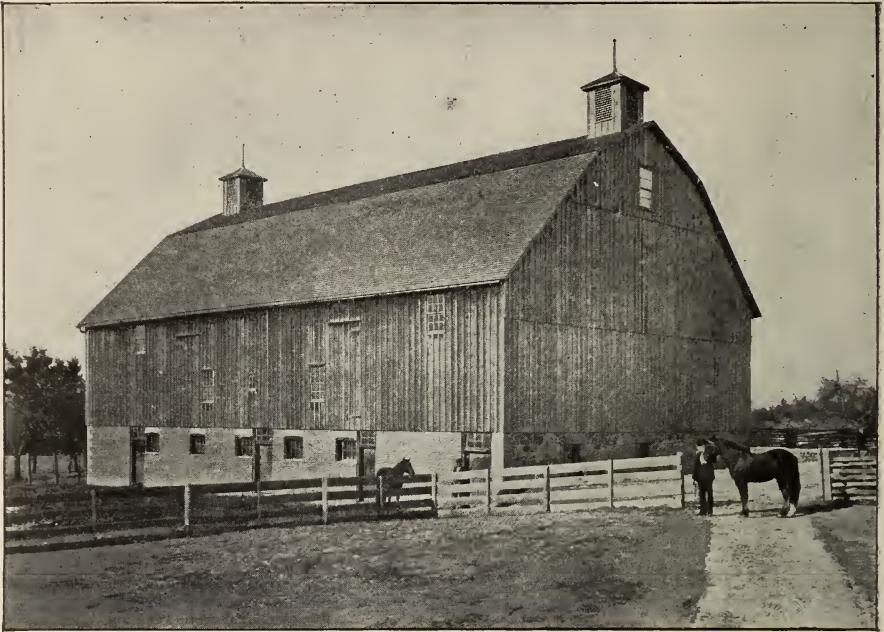
A MODERN BARN, With Basement Stable.
