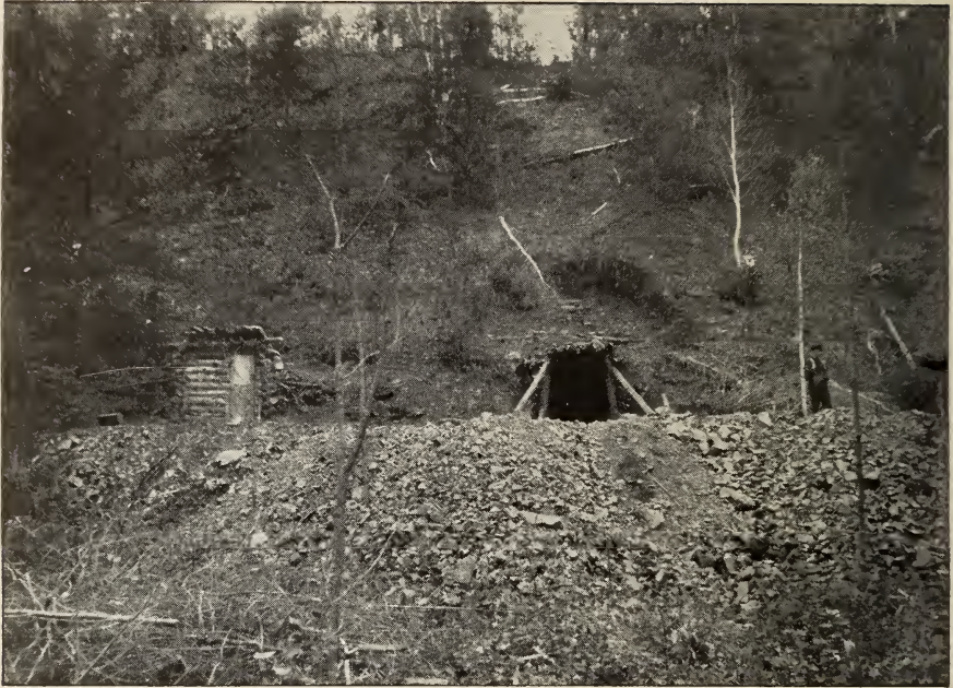
MOUTH OF TUNNEL, Atikokan Iron Range.
