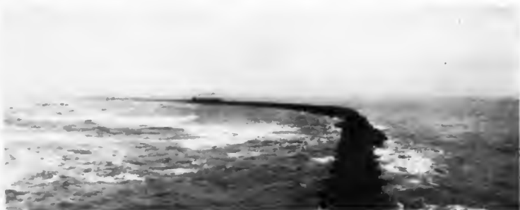
JETTY CONSTRUCTION AT MOUTH OF THE MAGDALENA
