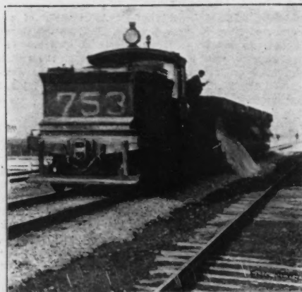
Fig. 5. Dumping Stone Ballast from Goodwin Cars, Illinois Central R. R.
