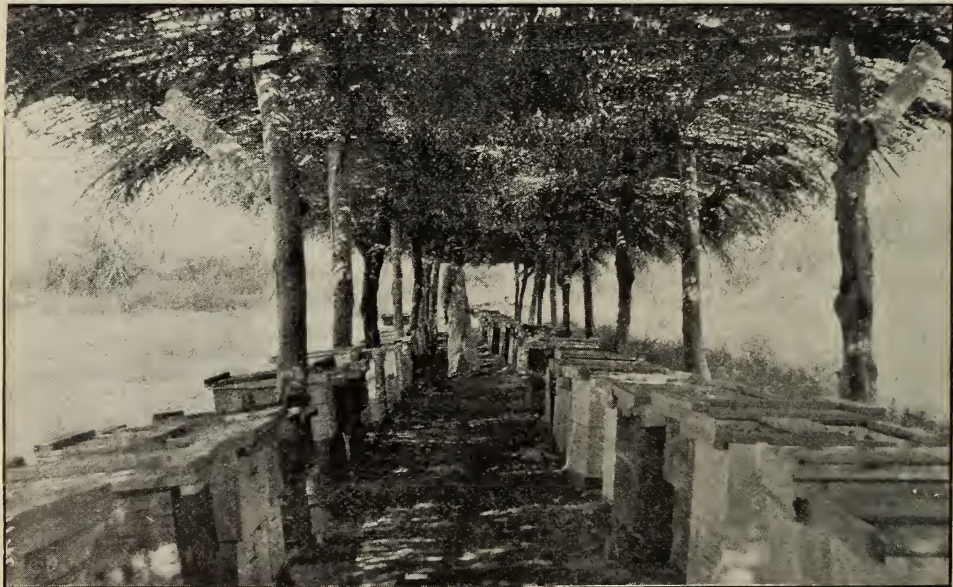
Bee-shed in Arizona, made by stretching wires across the tops of the posts and laying brush over them.
