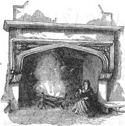
FIRE-PLACE—COBHAM HALL, KENT.
