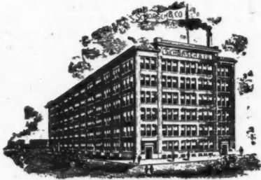
FACTORY 132 ND TO 133 RD ST. & BROOK AVE
