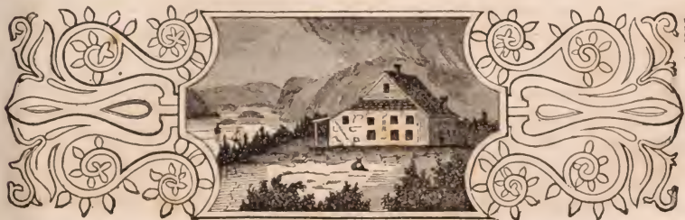
Washington's Head-quarters at Newburgh.
