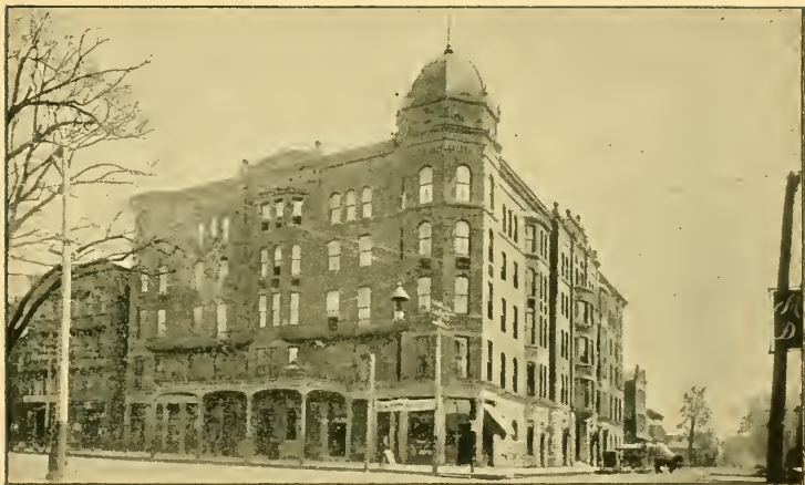
Ticket and Freight Offices, Burlington Route, Newcomb Hotel.
