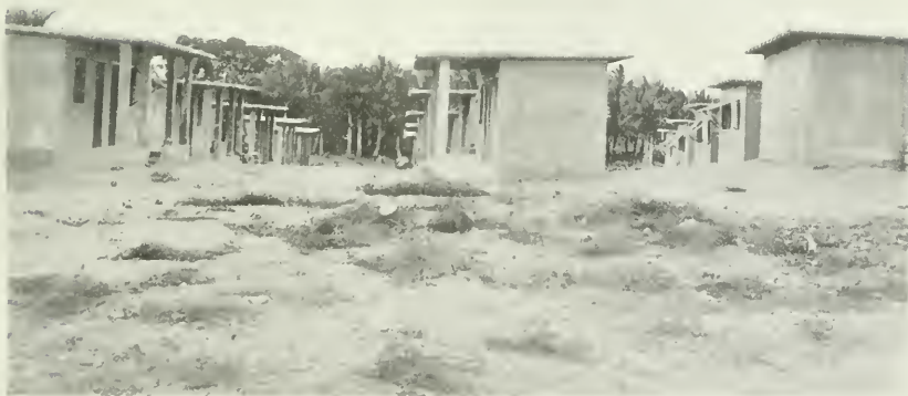
FIG. 4. CONCRETE DOUBLE COTTAGES FOR TWO LEPERS, LEPER COLONY, NIGUA, R. D.
