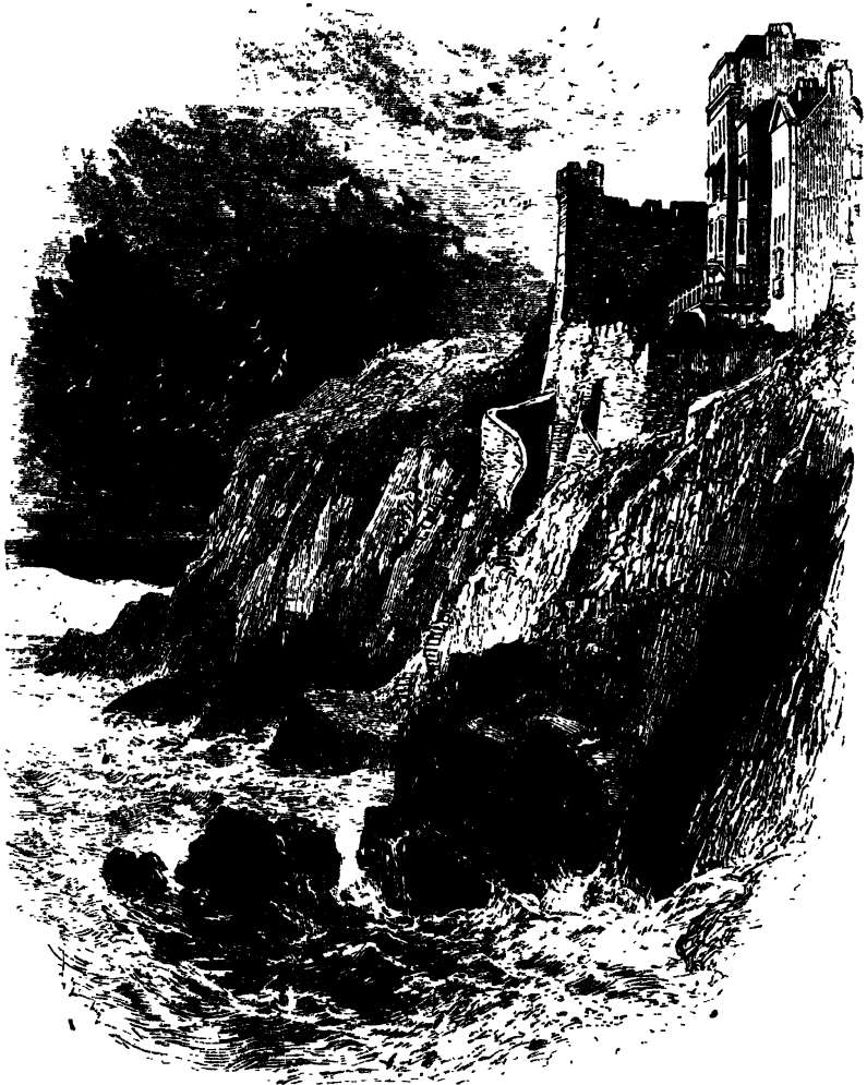
• TOWER ON THE SOUTH CLIFF.
