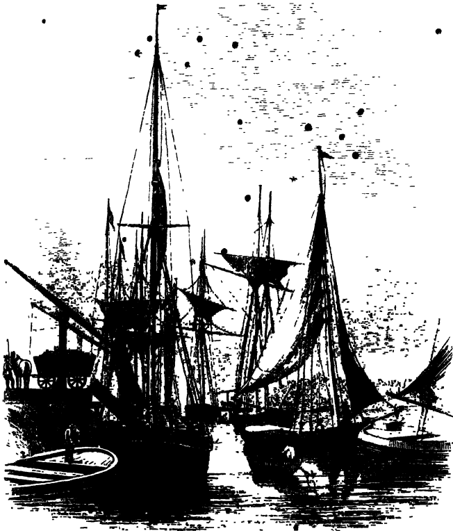
COAL BARGES AT LYDNEY.
