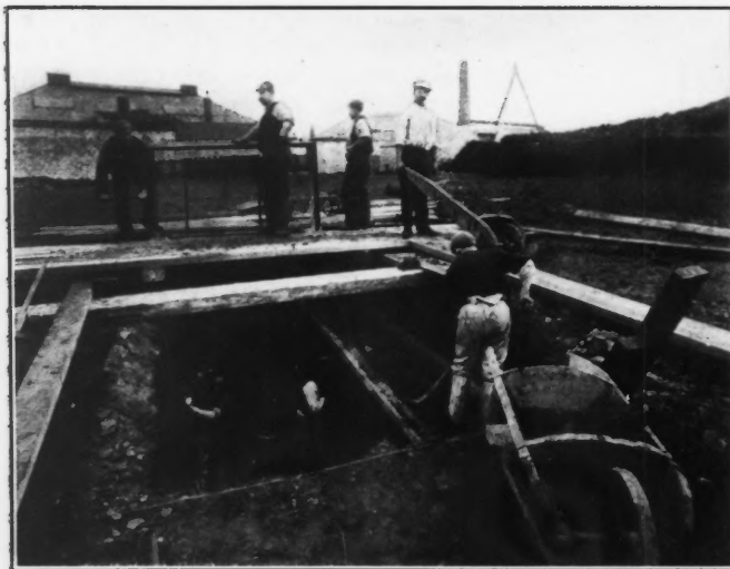
SINKING NEW SHAFT AT SOUTH CROFTY
