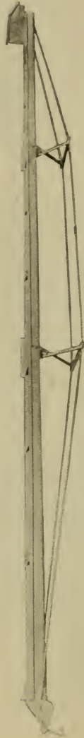
Ransome Forty-eight Foot Chute with Truss Members and Tension Rods in Position
