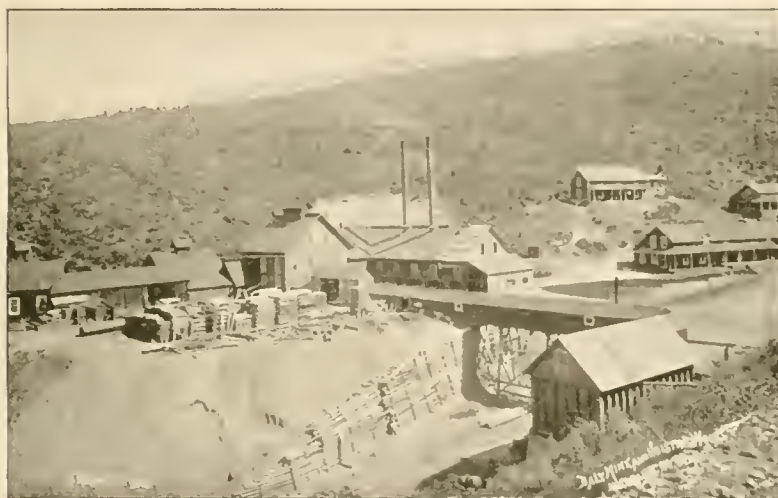
DALY MILLING AND HOISTING WORKS.
