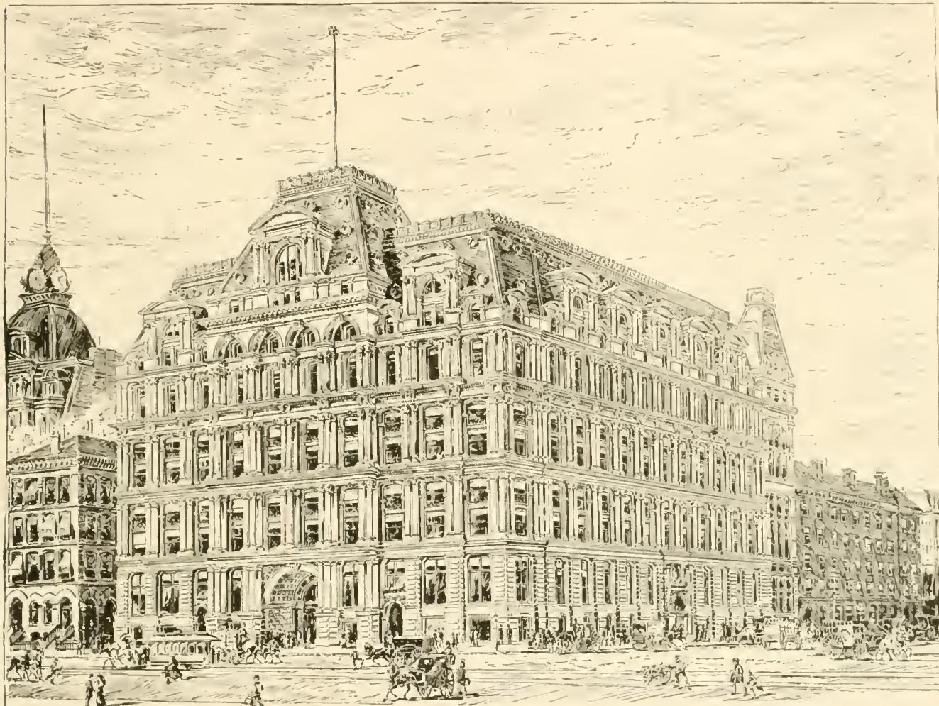
EQUITABLE LIFE ASSURANCE BUILDING, NEW YORK.
