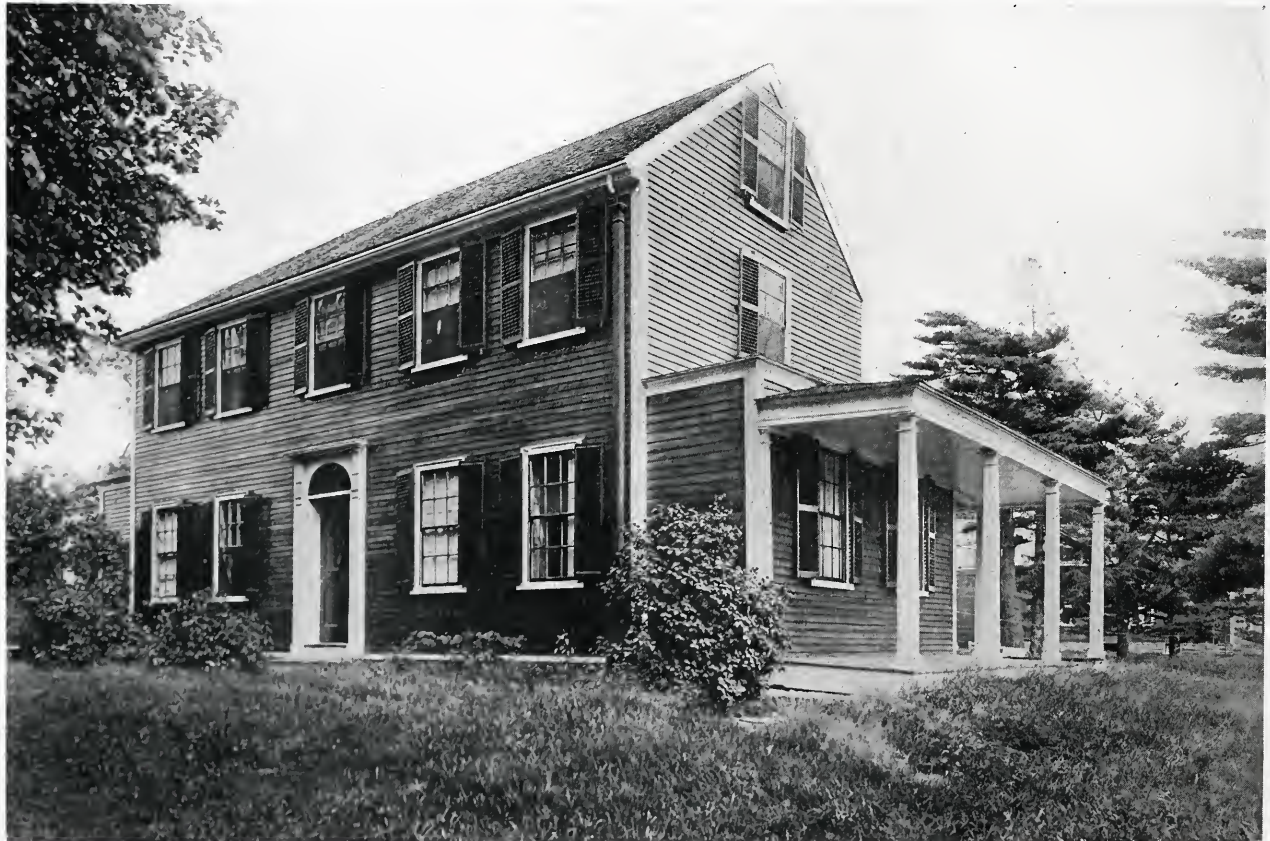
OLD FARM-HOUSE AT MILTON, MASSACHUSETTS. Built before 1800. An unusual element occurs in the old porch and in the projection of the first-story rooms.
