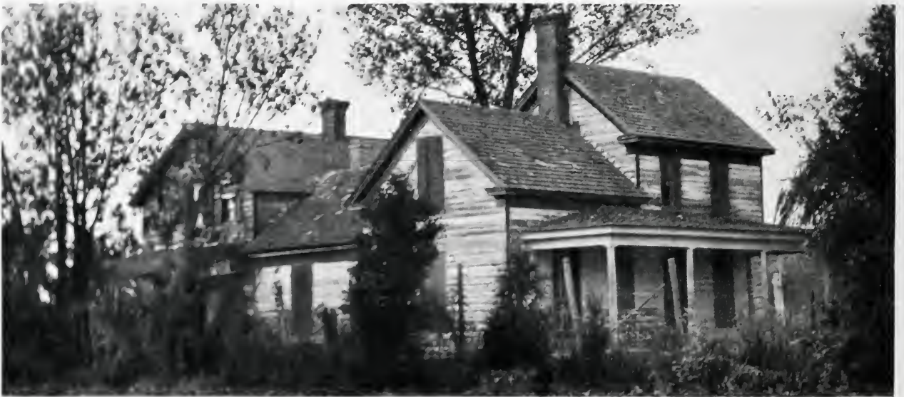
OLD HOUSE NEAR KINGSTON, MARYLAND.
