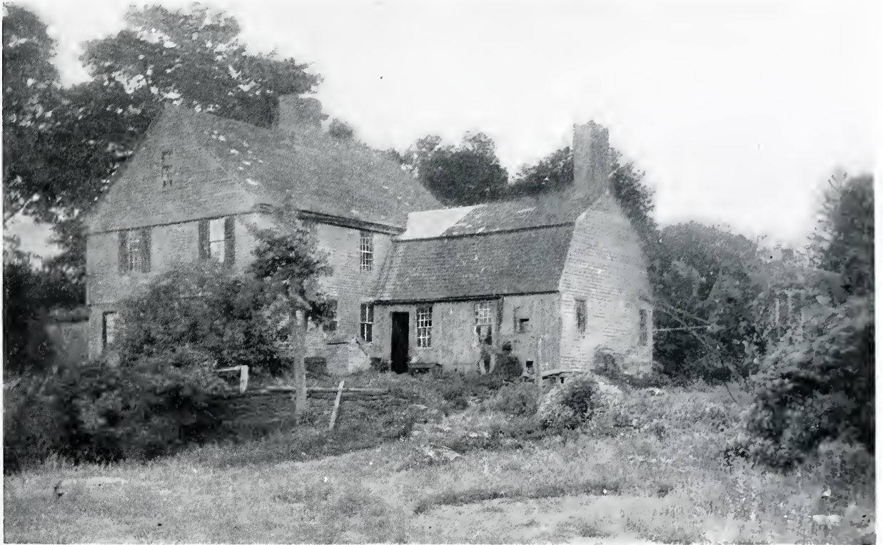
THE LOCKWOOD HOUSE, CROMWELL, CONNECTICUT. The main house is over two hundred years old. The gambrel-roofed ell composes nicely with the single-pitch roof of the house.
