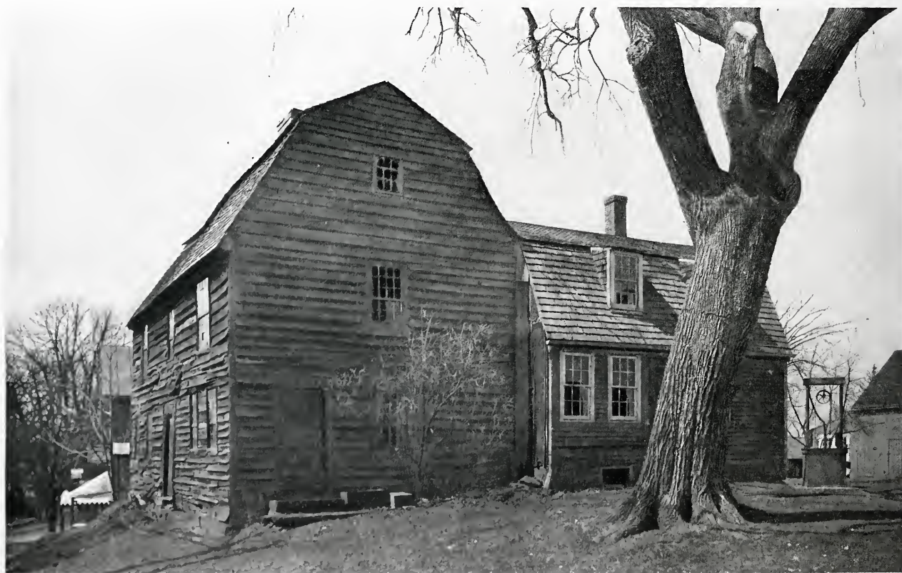
OLD HOUSE AT FARMINGTON, CONNECTICUT Gambrel of the third period with plan of the first period
