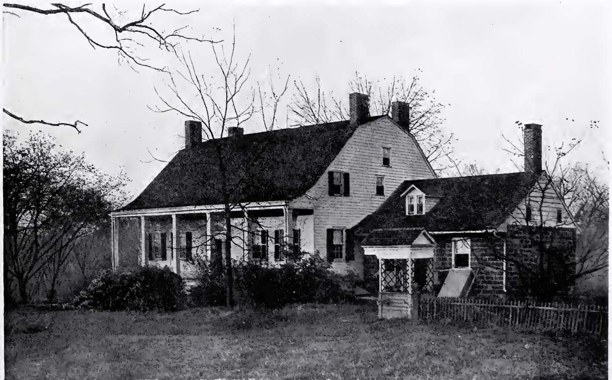
THE VREELAND HOUSE AT NORDHOFF, NEW JERSEY
