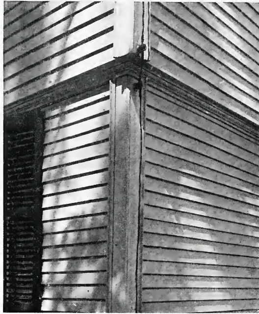
Detail of Corner Boards.
