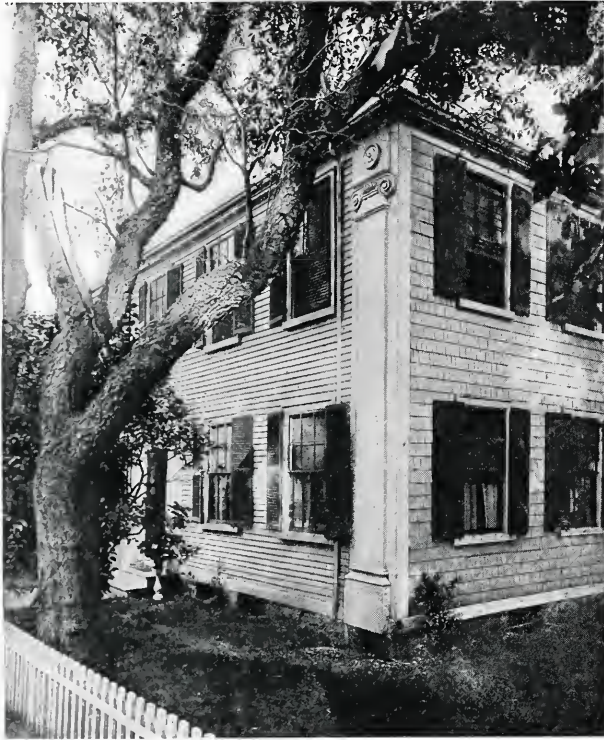
Detail of Pilaster.
