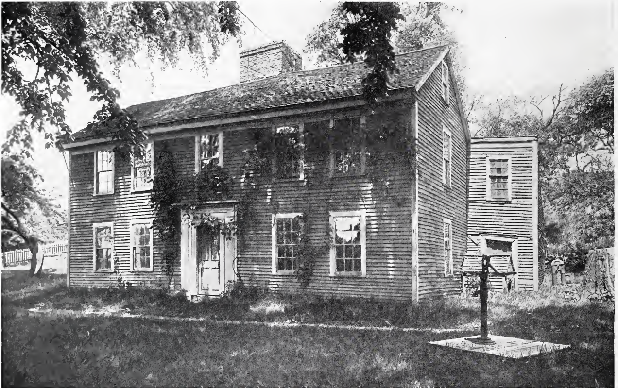
THE TYLER HOUSE AT WAYLAND, MASS. Built previous to 1725 A typical example of a farmhouse with a room on each side of entrance and a central chimney.
