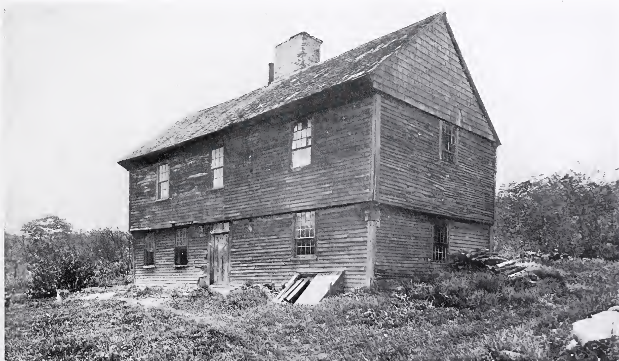
THE OLD BRAY HOUSE AT WEST GLOUCESTER, MASSACHUSETTS
