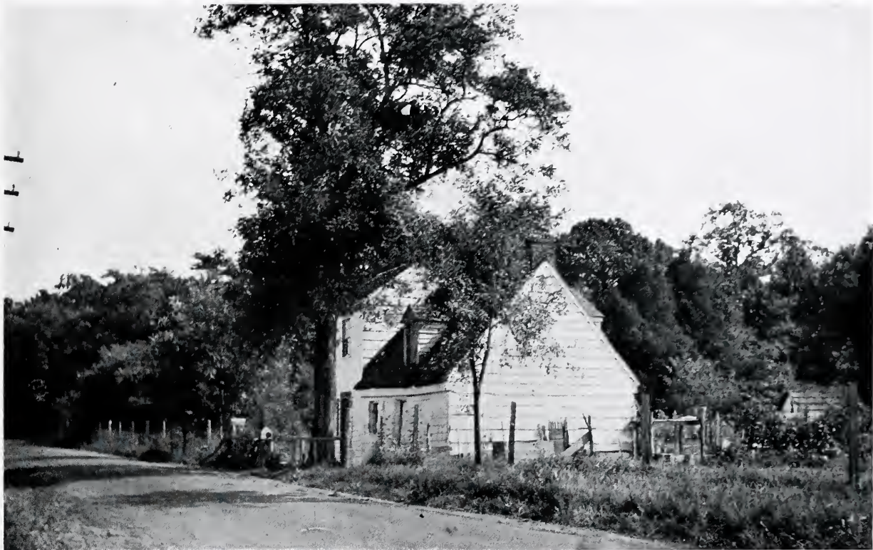
OLD HOUSE NEAR KINGSTON, MARYLAND
