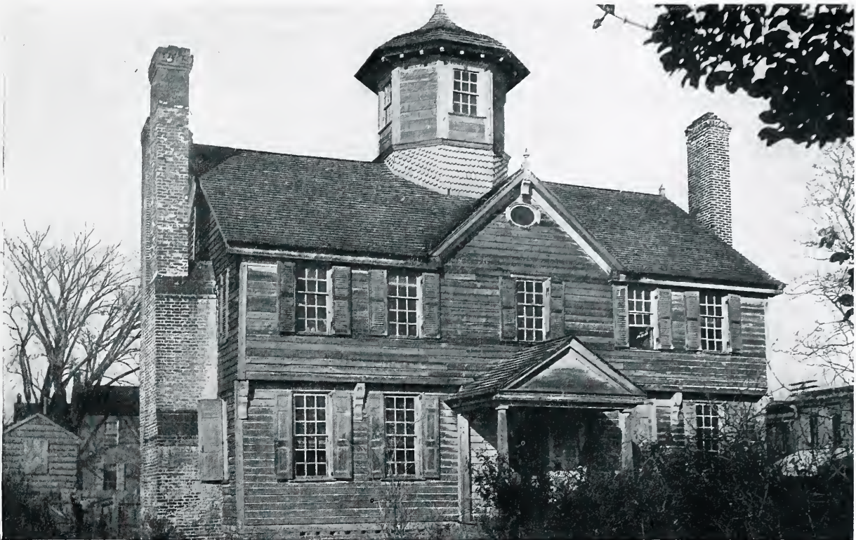
GOVERNOUR EDEN HOUSE, EDENTON, NORTH CAROLINA. Built about 1750 The framed overhang construction is most unusual in the Southern colonies
