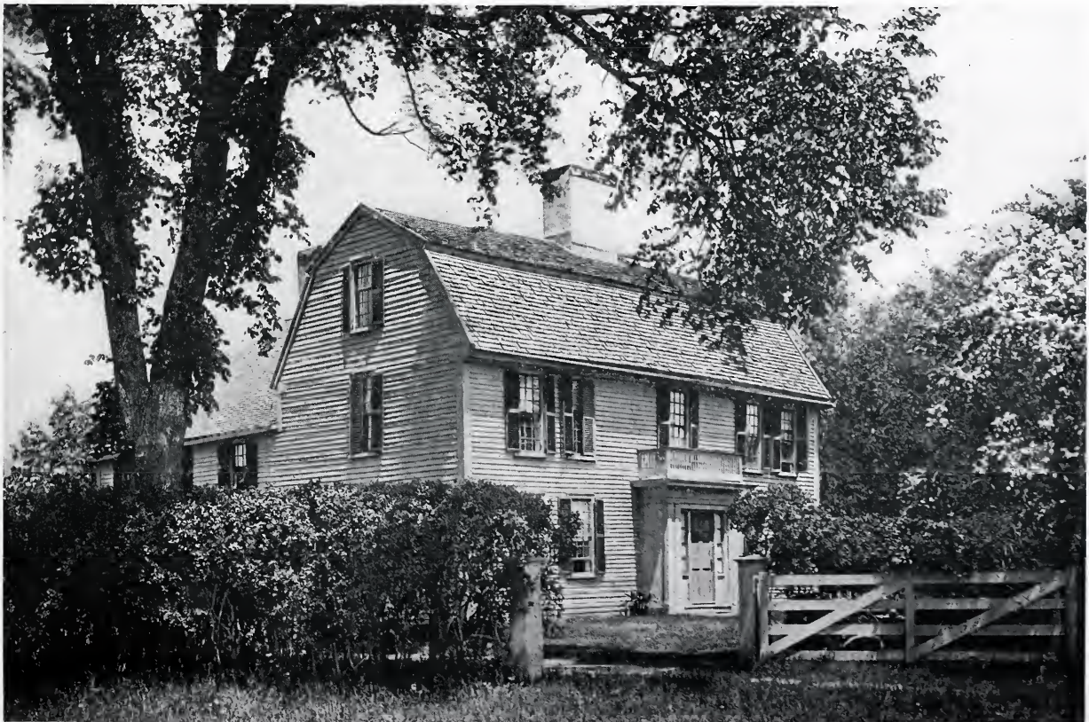
THE GENERAL PUTNAM HOUSE AT DANVERS, MASSACHUSETTS. Built about 1744. The outer vestibule and railing are carpenter additions.
