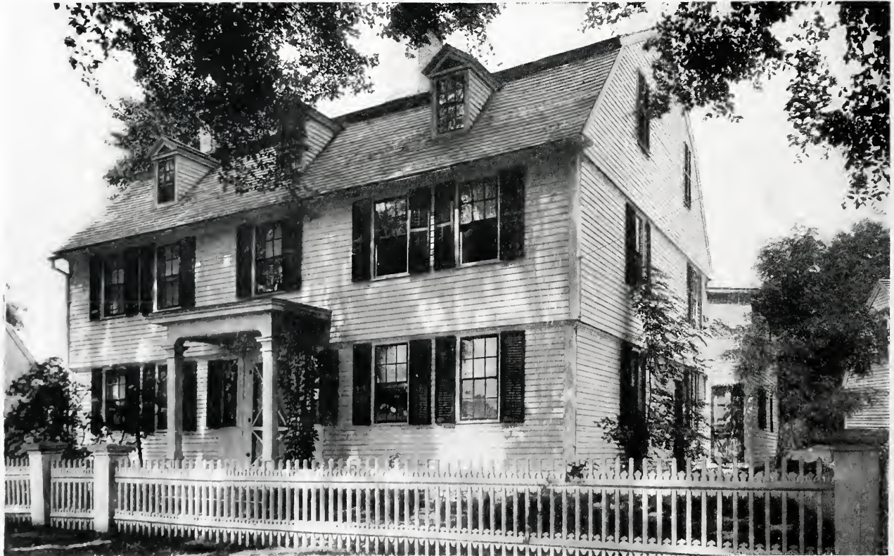
THE JABES BACON HOUSE, ON THE LOWER ROAD, WOODBURY, CONNECTICUT
