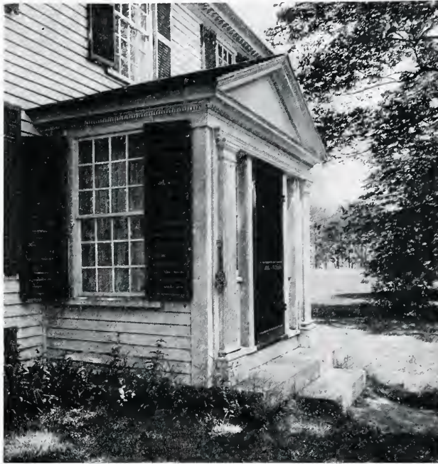
Detail, Entrance Vestibule.
