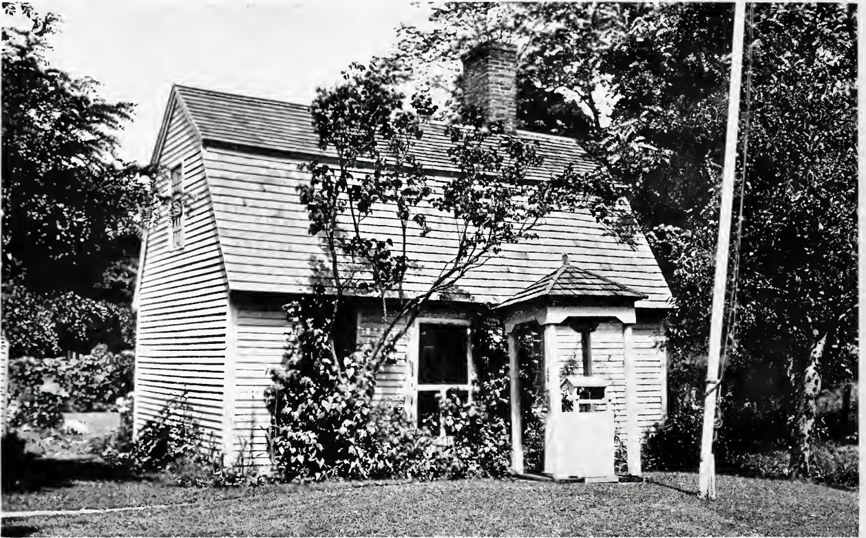
OLD SLAVE QUARTERS OF THE BACON HOUSE, WOODBURY, CONNECTICUT.
