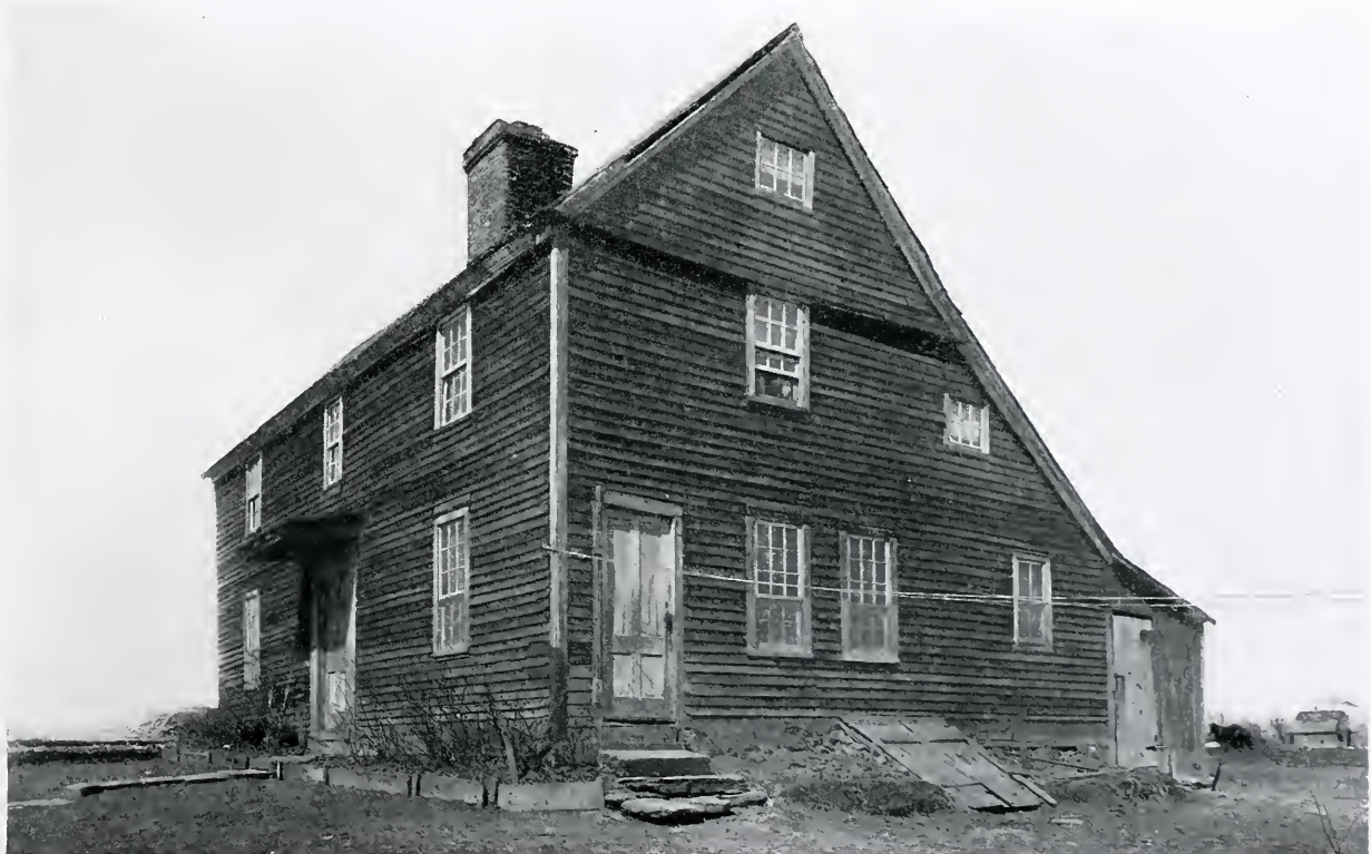
THE DEMING HOUSE, WETHERSFIELD, CONNECTICUT.
