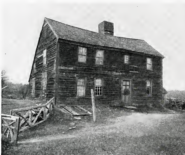
THE WAIT HOUSE, SOUTH LYME, MASSACHUSETTS. (?) Unsymmetrical placing of the windows.
