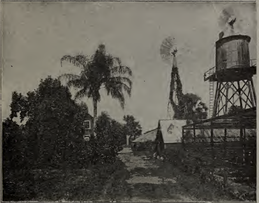
Water Tank, Greenhouses and Plant Packing House.
