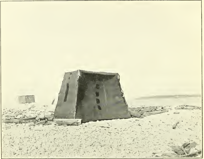
1. BLIND ERECTED ON MIDDLE STRAWBERRY ISLAND.
