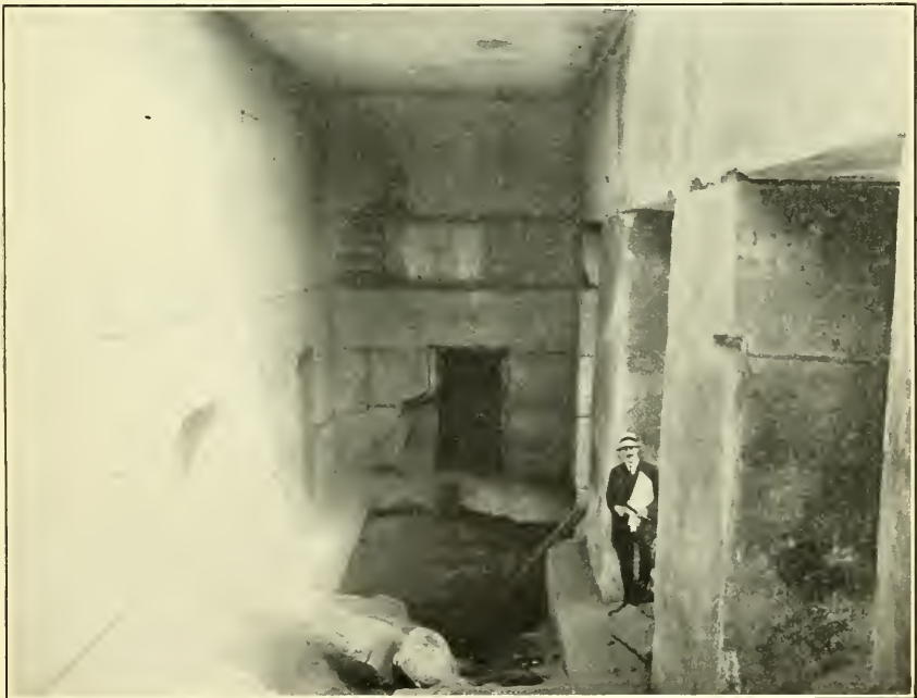
INTERIOR OF NORTHERN COLONNADE, SHOWING DOORS OF THREE CELLS; THE FOOT OF THE LADDER IN THE CORNER RESTS IN THE WATER OF THE POOL.
