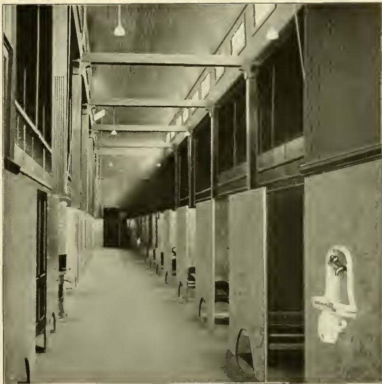
Interior of Bath Room, Baths of Arethusa
