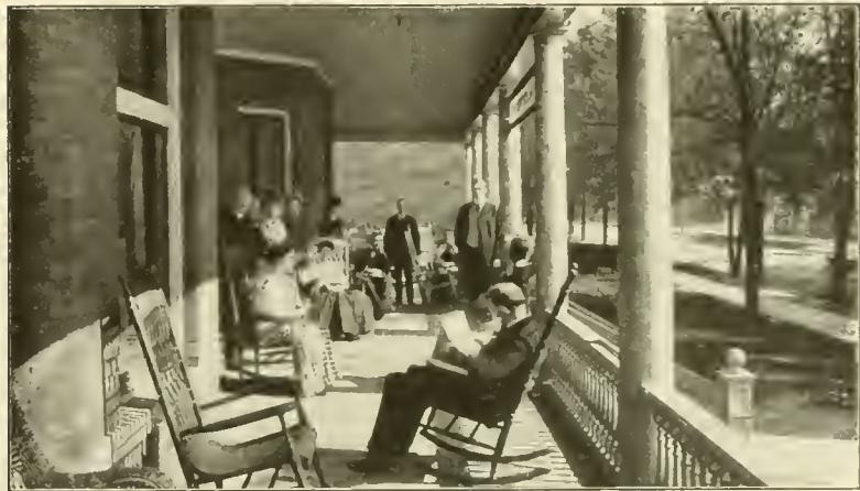
The Front Porch of the Glenwood
