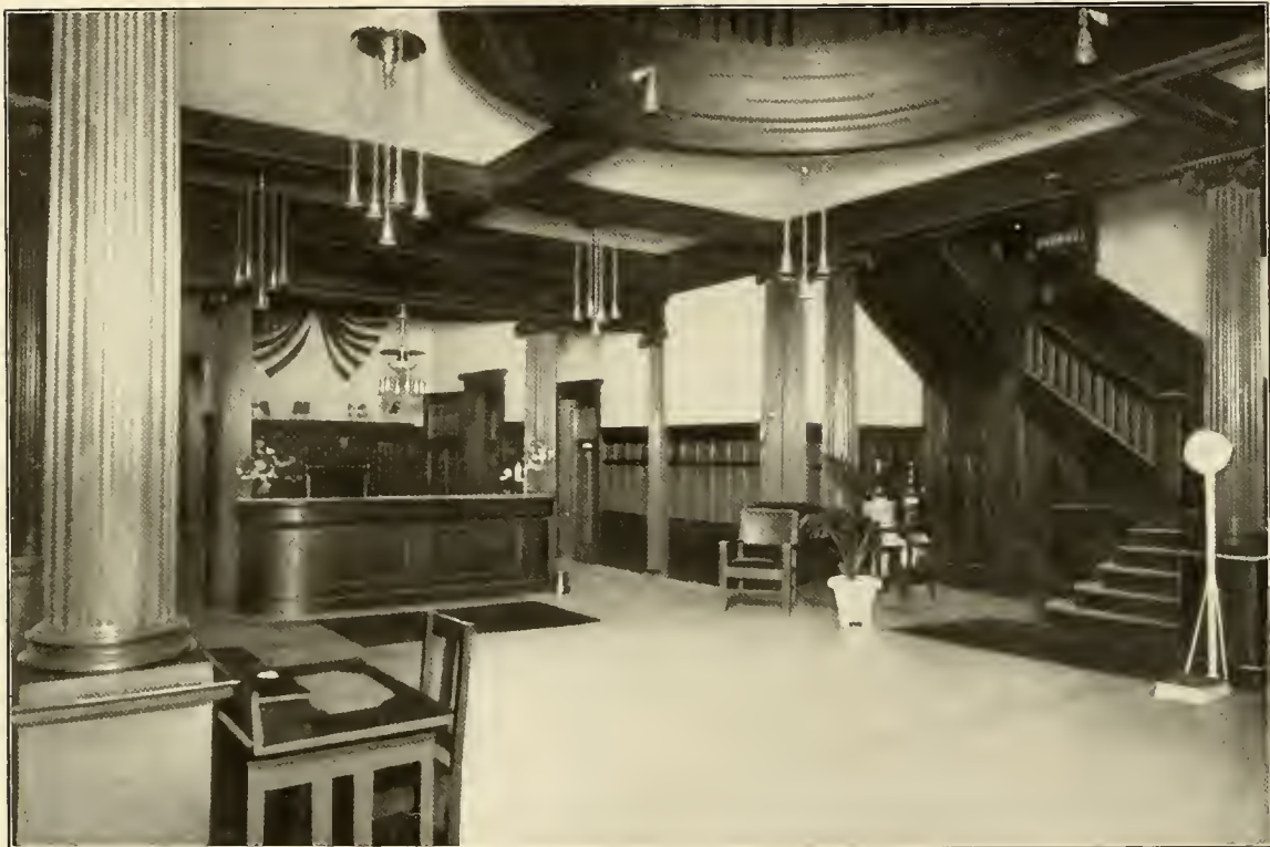
Lobby and Office of the Baths of Arethusa
