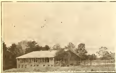
Above is shown one of the Mammoth laying and utility houses on the Sabrina Farm, Wellesley, Mass., this house is 60x60 feet a complete description of which we will give later for it is one of the most practical houses we have ever seen. In the basement are the incubators, cold storage department, etc. Another house just like this is now being built.—H. P. S.
