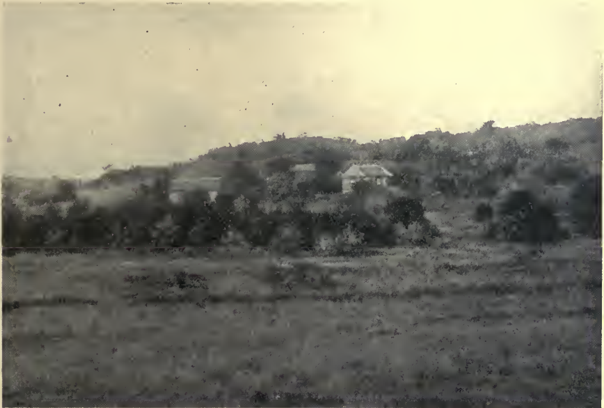
THE BUILDINGS OF THE DEFUNCT INDUSTRIAL INSTITUTION AT HOPE FOUNTAIN.
