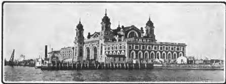
The Buildings, as they appear from the Bay
