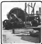
The Engine which raised the Cables
