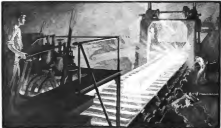
Rolling large "I" Beams for Structural Iron-Work
