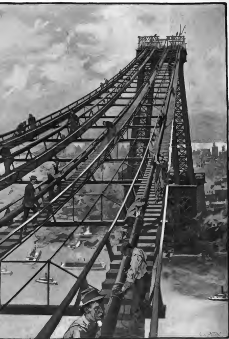
METHOD OF WRAPPING THE CABLES OF THE NEW EAST RIVER BRIDGE
