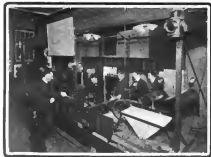
Explaining the Electrical Details
