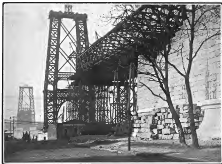
General View of the Structure from the Williamsburg Side
