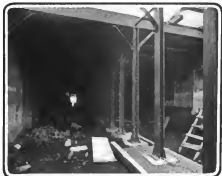
A completed Section at 135th Street and Broadway
