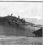
Building the Dem
