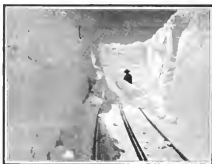
Clearing the Road
