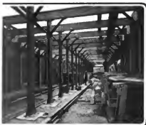
A Section ready for Roofing In
