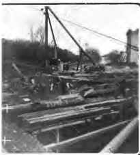
Covering in the Structure at 110th Street and Lenox Avenue
