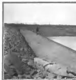
The Mud Dock, Completed
