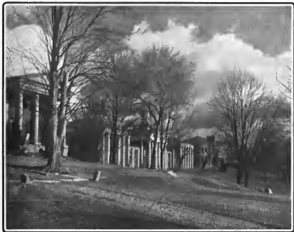
Main Buildings of Washington and Lee University,—Tucker Memorial Hall on the Right
