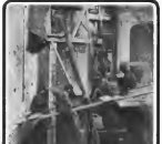
Coming up out of the Caisson
