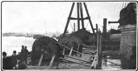
The Scow with the Cable-spools starting across the River, April 10
