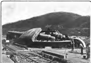
Assembling a Groson Turret
