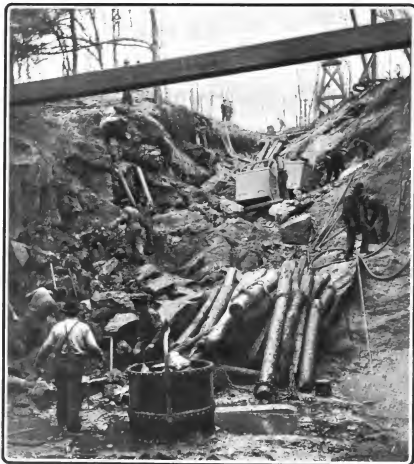
DIGGING THROUGH CENTRAL PARK ALONG THE LINE OF THE UNDERGROUND RAILROAD
