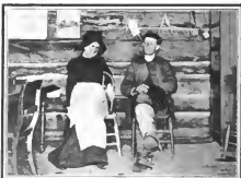
Mrs. Howe, the only Occupant of the Section-House near the Summit, and Engineer McCaul
