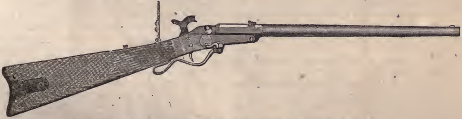
MAYNARD RIFLE.—Fig. 1. Showing Rifle loaded, cocked, and with back sight raised.
