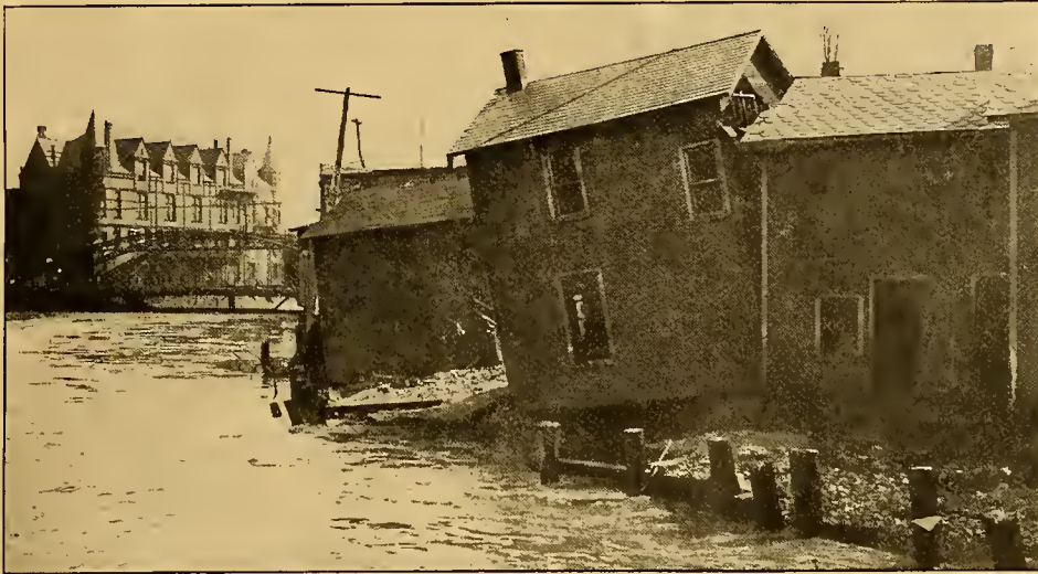
HOUSES TILTED IN REAR OF PORTER STREET
