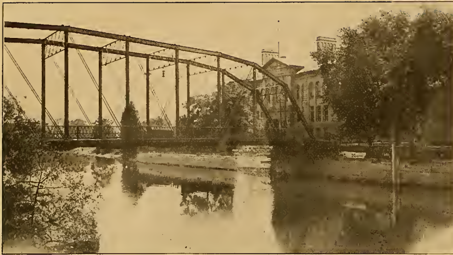
CHESTNUT STREET BRIDGE AT LOW WATER
