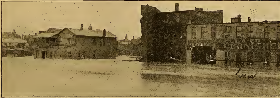
SHOWING GAP IN BELL & CO. WALLS AND HERALD WALL
