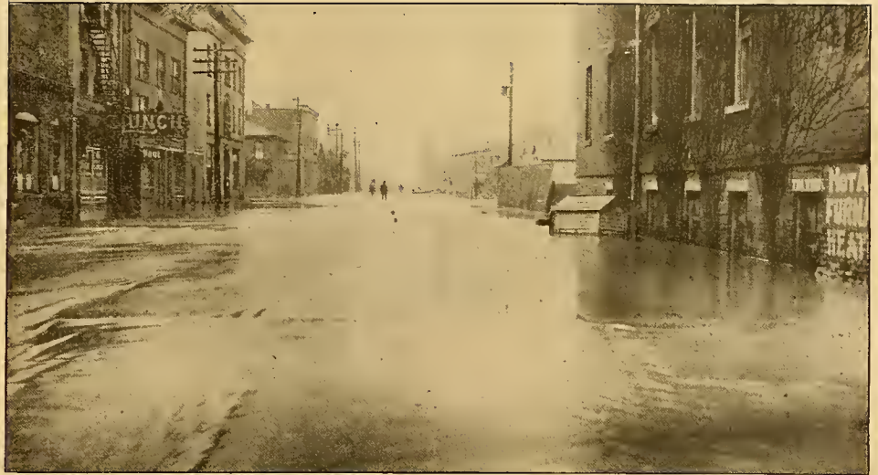
P. R. R. TRACKS SUBMERGED ON RAILROAD STREET
