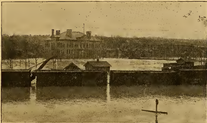
PENNSY TRACKS UNDER WATER —Photo by Heintz
