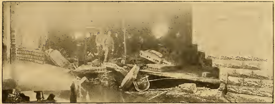
WRECK OF AUTO GARAGE ON CHESTNUT STREET —Photo by Cubbison
