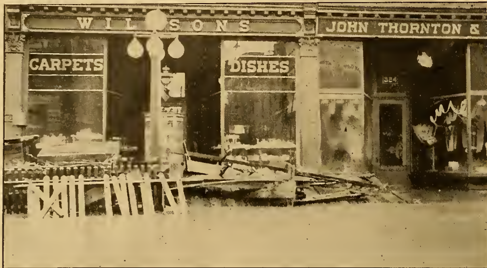
DEBRIS IN FRONT OF STATE STREET STORES
