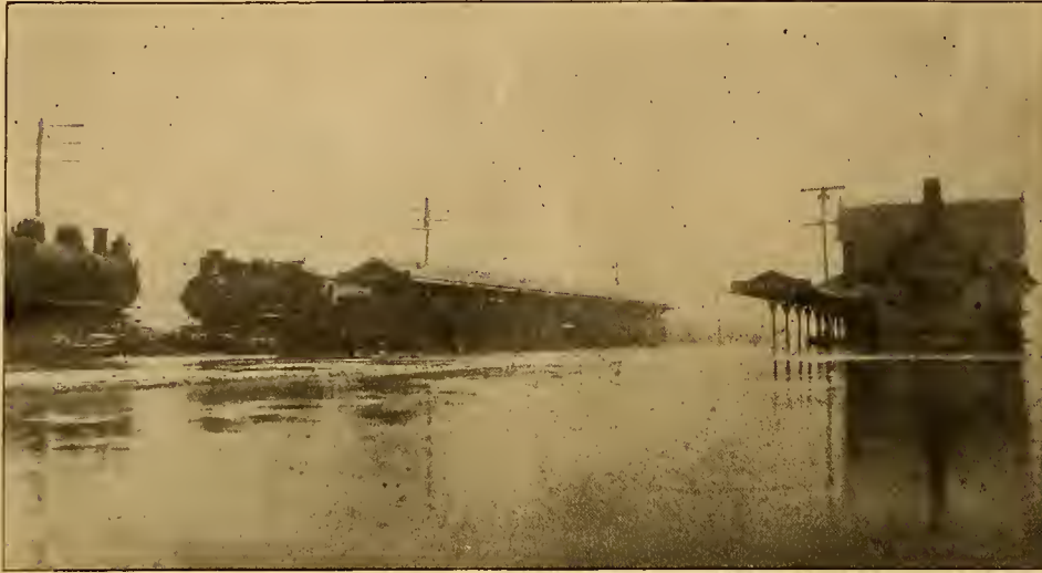
PENNSY STATION AND STALLED TRAINS IN WATER
