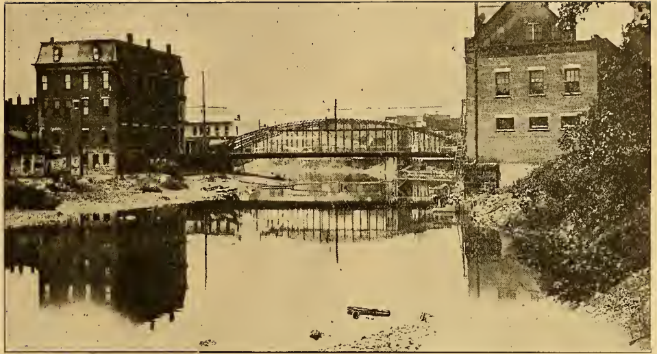
STATE STREET BRIDGE AT LOW WATER
