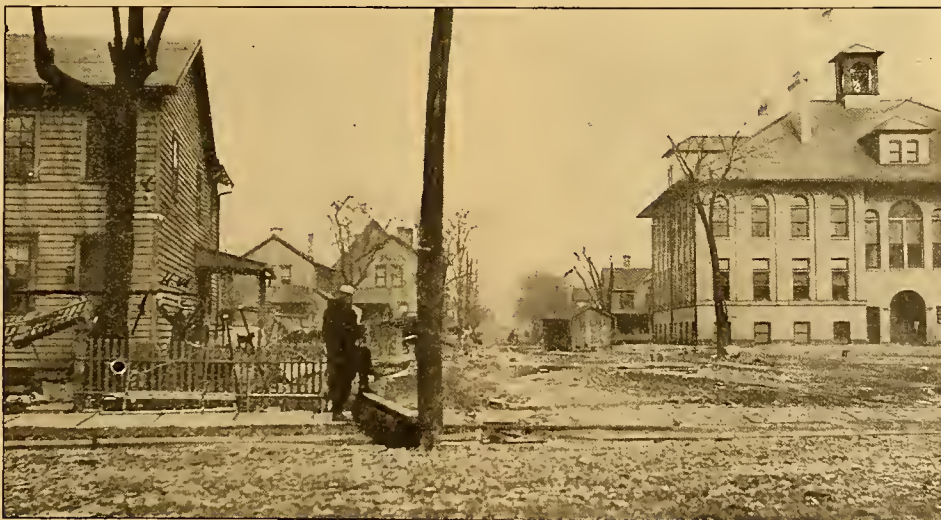
HIGH WATER MARK NEAR CENTRAL SCHOOL
