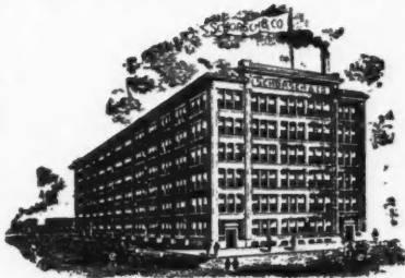
FACTORY 132 ND TO 133 RD ST & BROOK AVE
