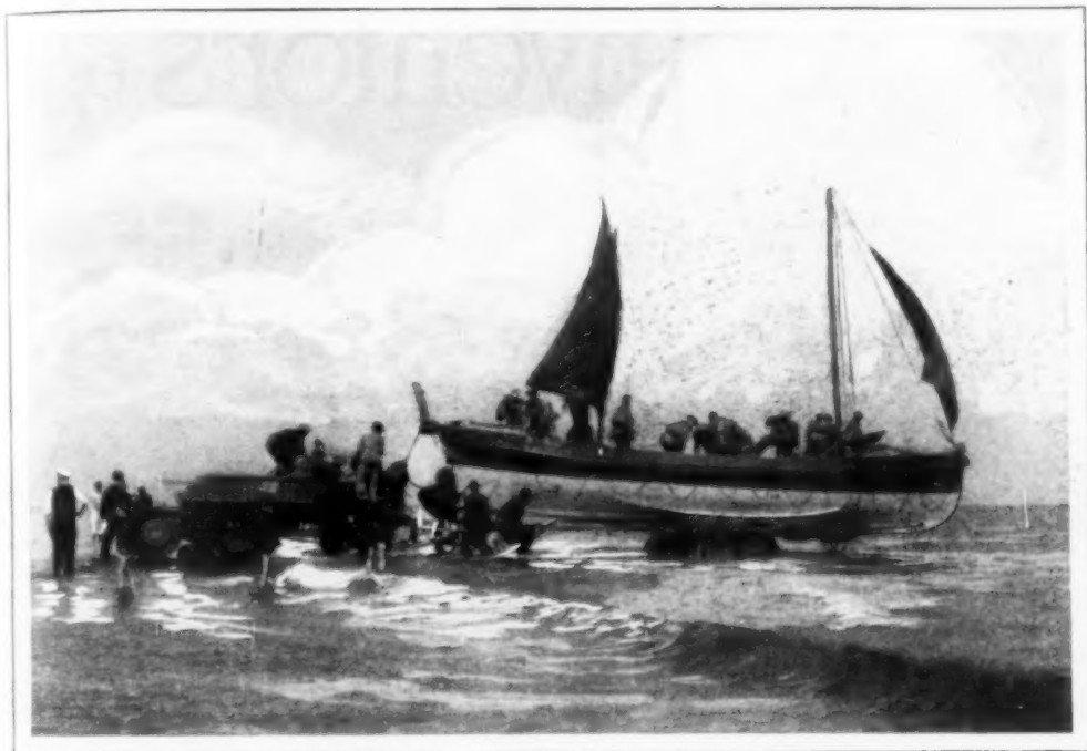
Launching the Big Lifeboat with Aid of Tractor That Hauls It across Sands and Rough Shore, Pushes It into the Water and Hauls It Out Again
