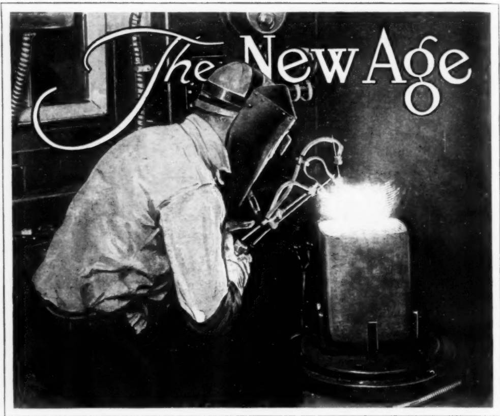
The Latest Thing in Electric Welding, the Atomic-Hydrogen Process; Hydrogen Fed to the Arc Has Its Molecules Broken into Atoms, Which, in Recombining, Produce Intense Heat
