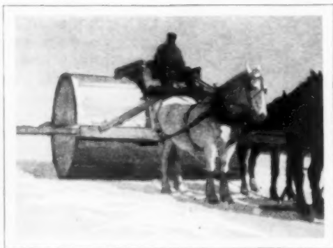
Packing the Snow with Big Roller Instead of Shovel It Away; How Roads Are Kept Clear in Colorado
