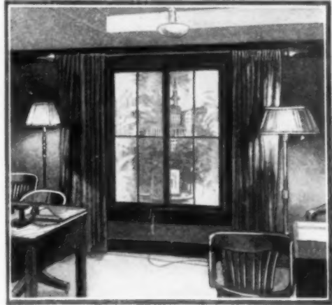
False Window with Electrically Lighted Background, to Give Outdoor Appearance to Basement Room
