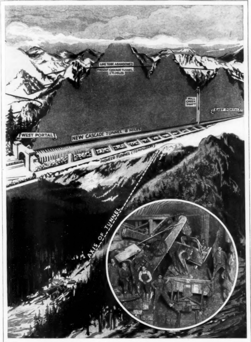
Cross Section of the Cascades, Showing the New Tunnel 500 Feet Below the Present Railroad Line; Photograph of the Range under Which the Big Bore Passes, and, in Circle, One of the Compressed-Air Shovels That Works in Limited Quarters to Clear Away the Rock
