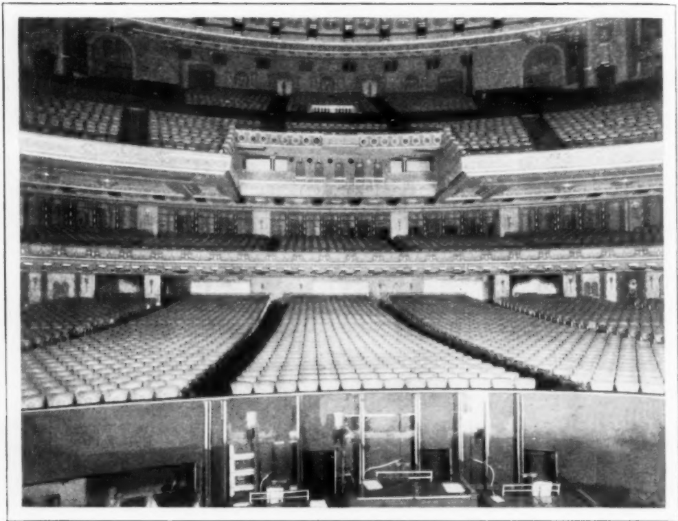
How a Huge Theater Looks from the Wings; the Orchestra Pit Has Been Lowered to the Basement; the Cut-Away Section of the Upper Balcony Shows Spotlights and the Movie Booths
