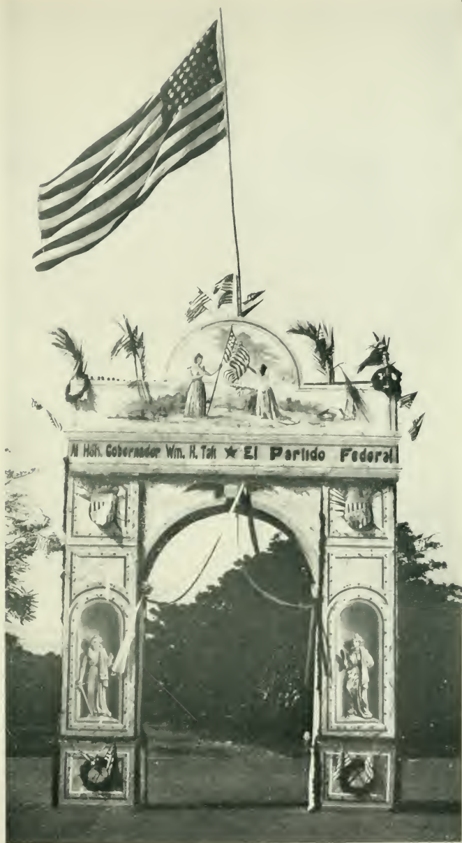
ARCH ERECTED BY THE PARTIDO FEDERAL REPRESENTING FILIPINA OFFERING ANOTHER STAR TO THE AMERICAN FLAG
