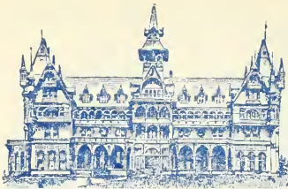
PERALTA HALL, BERKELEY, CAL.
