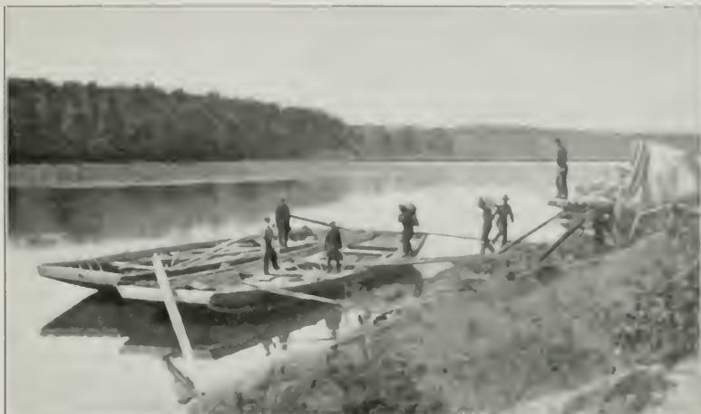
Loading trial shipment of bituminous sand from point on east side Athabaska river, 5 miles below McKay.
