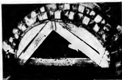
FIG. 127. —Centering for Brick Sewer.
