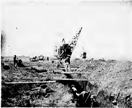
FIG. 94.—Drag Line at Work on Trench for Drain Tile.
