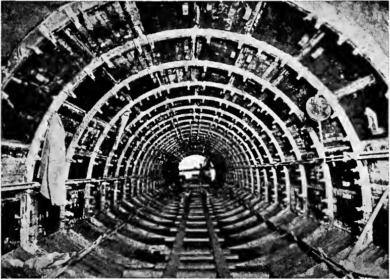
FIG. 139.—Interior of Steel Forms for Calumet Sewer, Chicago.
