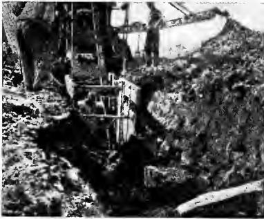
FIG. 91.—Movable Sheeting Fastened to Traction Ditcher.
