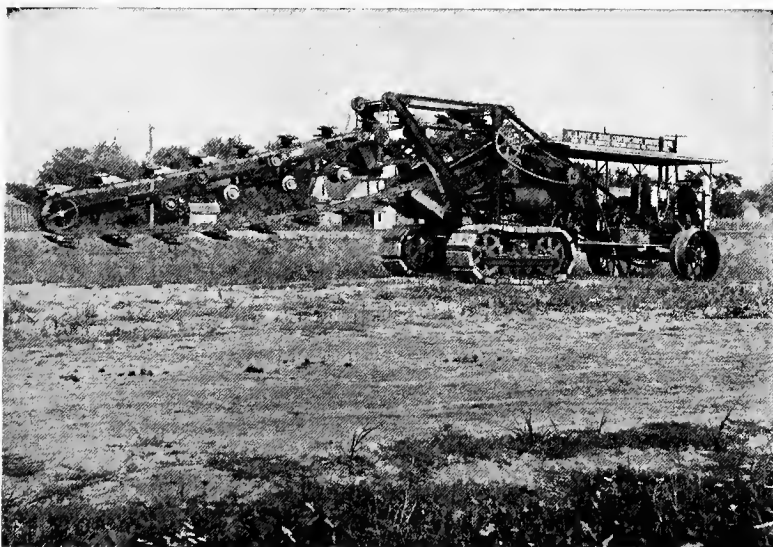
FIG. 90.—Buckeye Endless-chain Excavator. Courtesy, Buckeye Traction Ditcher Co.
