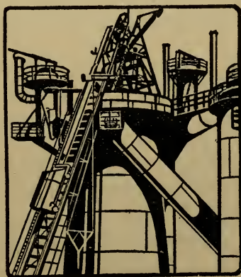
TOP OF BLAST FURNACE SHOWING METHOD OF FILLING
