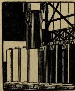
STRIPPING THE MOLDS FROM THE INGOTS
