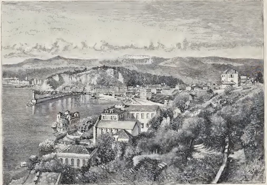
No. 37.—Nice from above the New Villefranche Road. Engraved by J. C. Griffiths.
