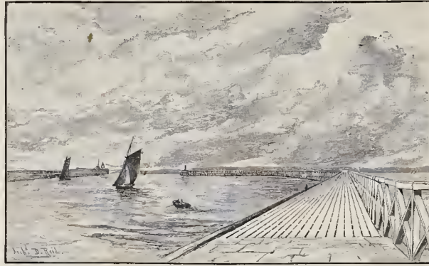
No. 2.—The East Pier, Leith. Engraved by H. S. Percy.
