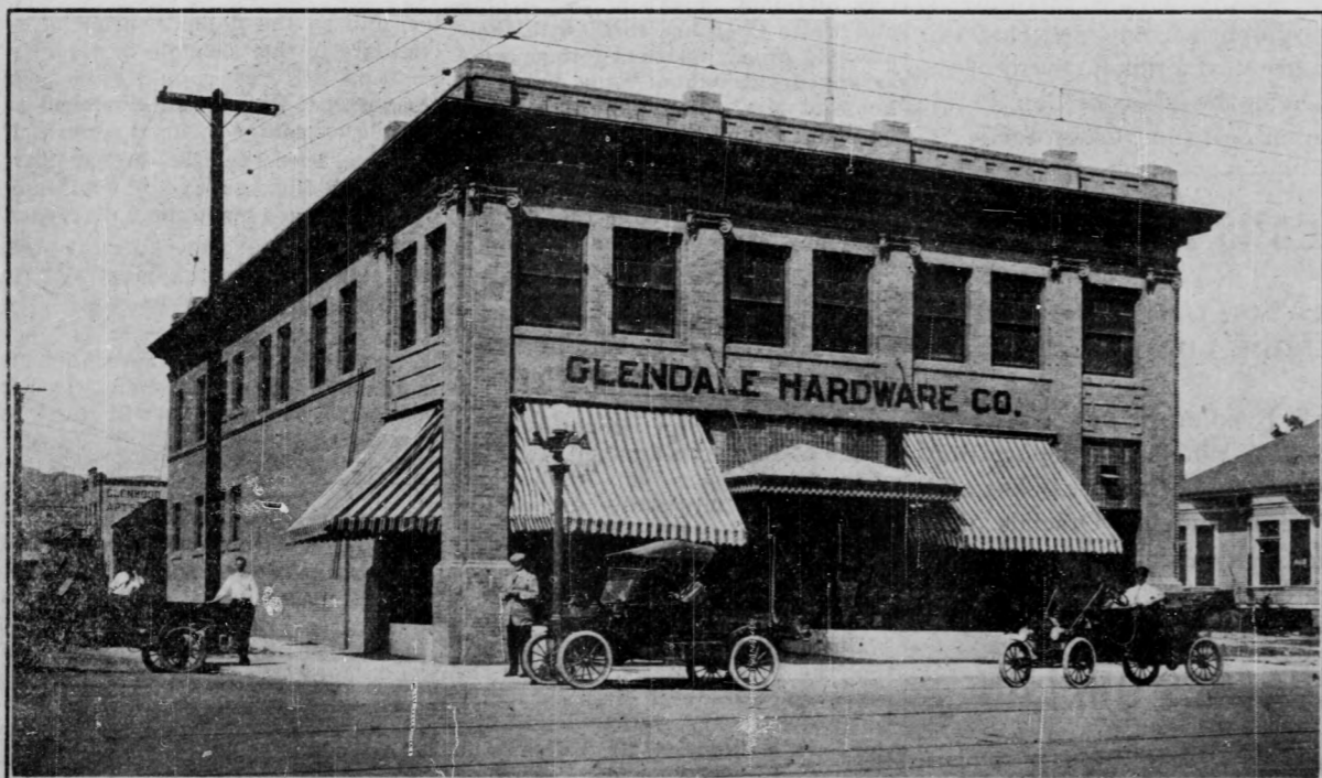
Glendale Hardware Building, Corner Broadway and Isabel
