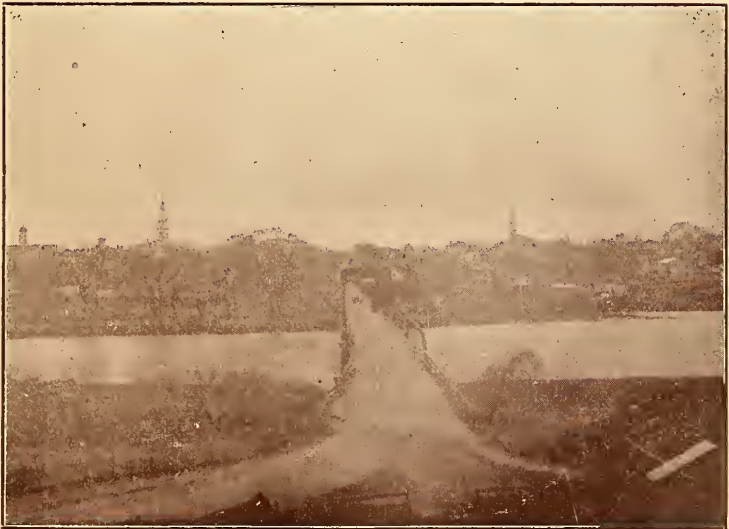
View of Fredericksburg from Stafford Heights, where Federal guns were located in 1862, showing the old Scott bridge.
