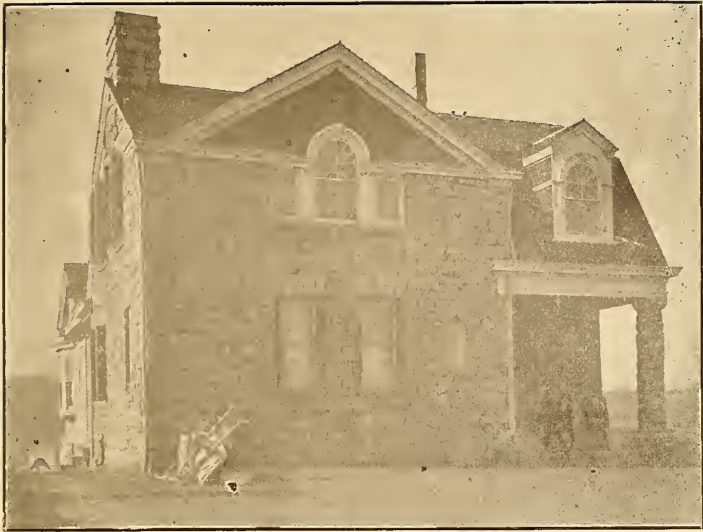
“The Lodge” at Mary Washington Monument. Constructed of Virginia Granite for Superintendent of Monument and Grounds. (See page 160)
