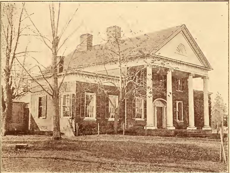
"Marye Mansion," Gen. Longstreet's headquarters at Battle of Fredericksburg, December 13, 1862; now the residence of Capt. M. B. Rowe.
