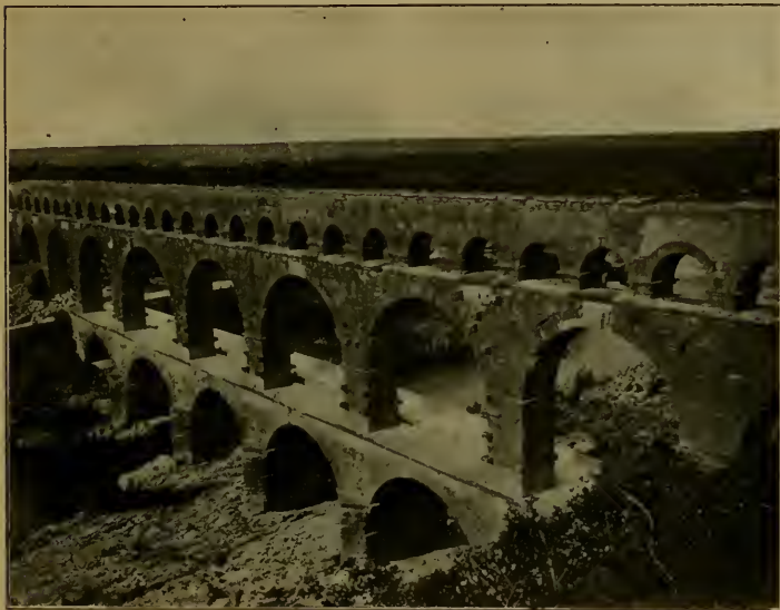
ROMAN AQUEDUCT NEAR NÎMES, FRANCE: present condition. — From a photograph. This structure was built by the Emperor Antoninus Pius, about 150 A.D., to bring water from distant mountain springs. Some of these Roman aqueducts remained in use until recent days.
