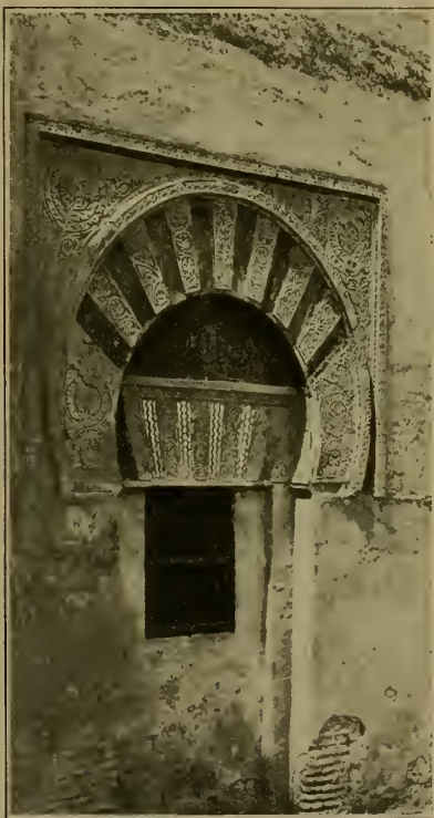
A WINDOW IN THE MOSQUE AT CORDOVA. See also p. 40 for Mohammedan architecture.
