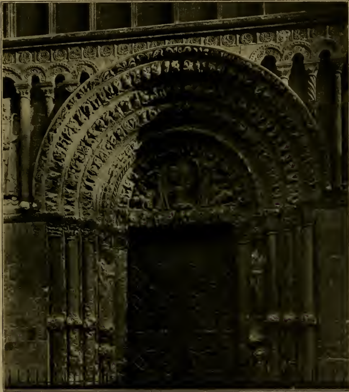
A NORMAN DOOR IN CANTERBURY CATHEDRAL. — Note the massive round arch and the simple but effective ornament.
