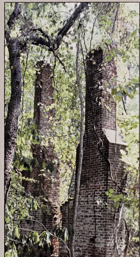
The Chiles home site (mid-1700s) is just one of the historical, archaeological, and architectural properties managed by Eastern States along the Potomac River in Maryland and Virginia.
