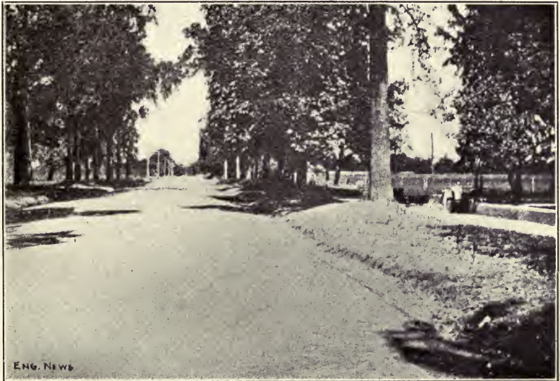
FIG. 4.—MACADAM ROAD WITH SHALLOW DITCHES. (Showing macadam (6 ins. x 16 ft.) road without ditches; earth shoulders 7 ft. wide; crown of road 15 ins. above bottom of earth gutter.)
