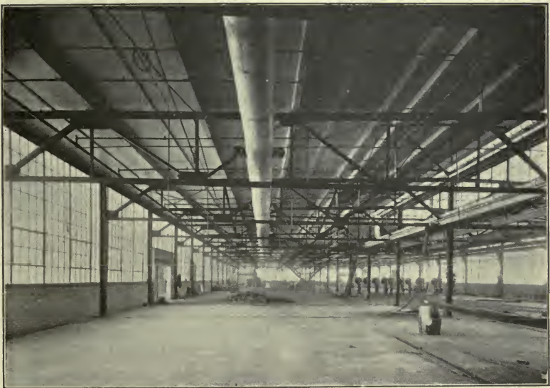
FIG. 21.—Hot blast heating system as applied to shop of the Jaxon Steel Products Co., Jackson, Mich. Courtesy of the Austin Co., Cleveland, Ohio.
