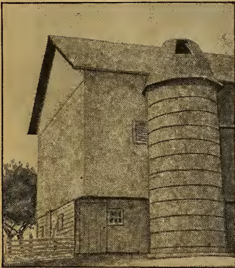
Building this 50-ton silo was mostly a one-man job
