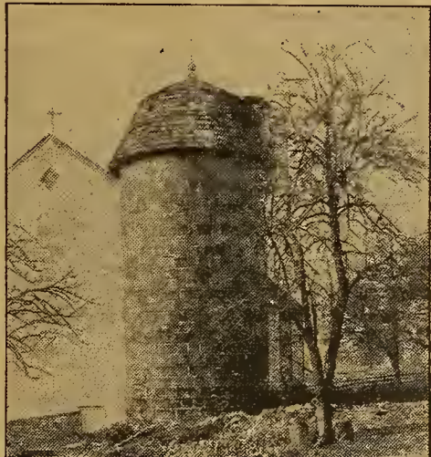
The high roof of this silo enables it to hold more silage, and even after settling, the silage is about level with top of wall
