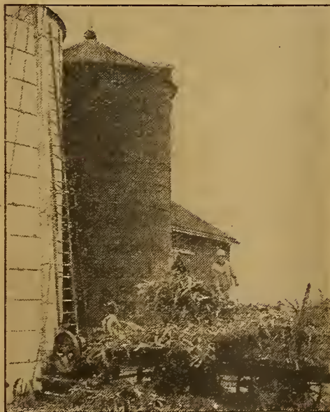
Silos with low roofs require refilling if they are to hold their full capacity.
