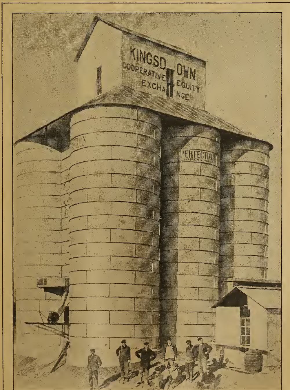
This is one of many similar farmers' elevators in the Middle West. It has all modern equipment, is fire-proof, and has a capacity of 30,000 bushels
