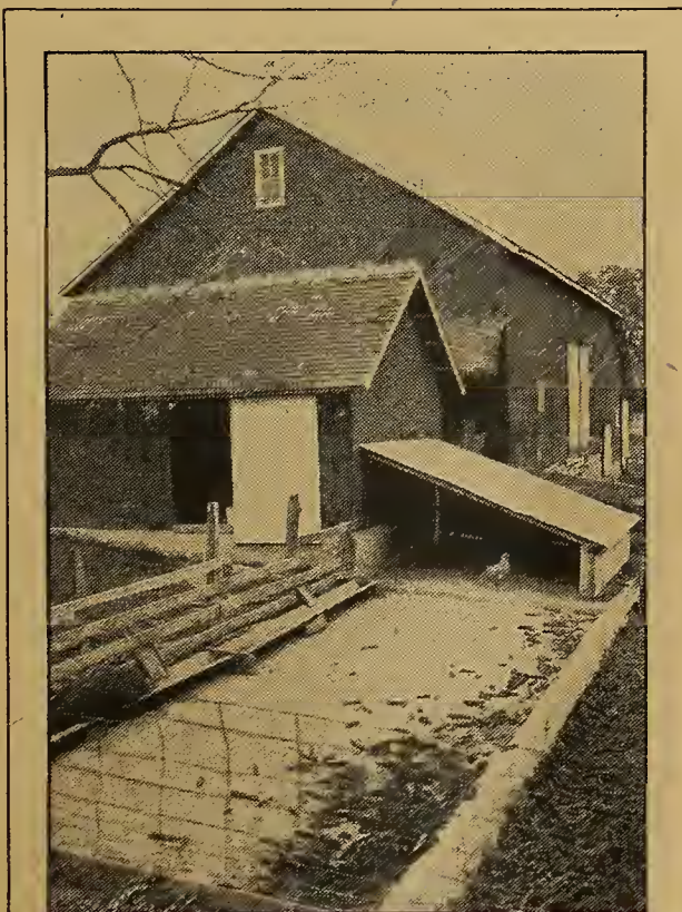
Concrete feeding floors prevent waste of corn and keep hogs cleaner
